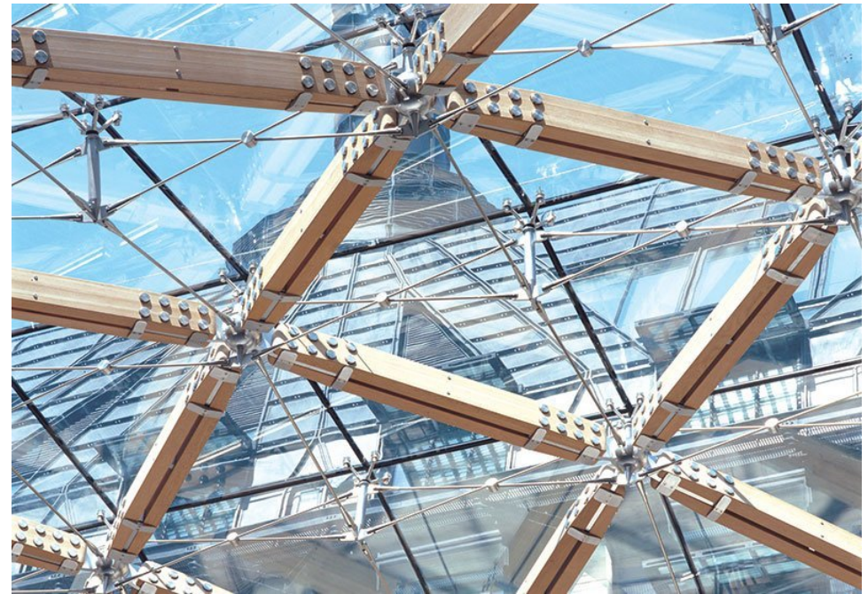
Figure 27: Portcullis House gridshell by Hopkins Architects
