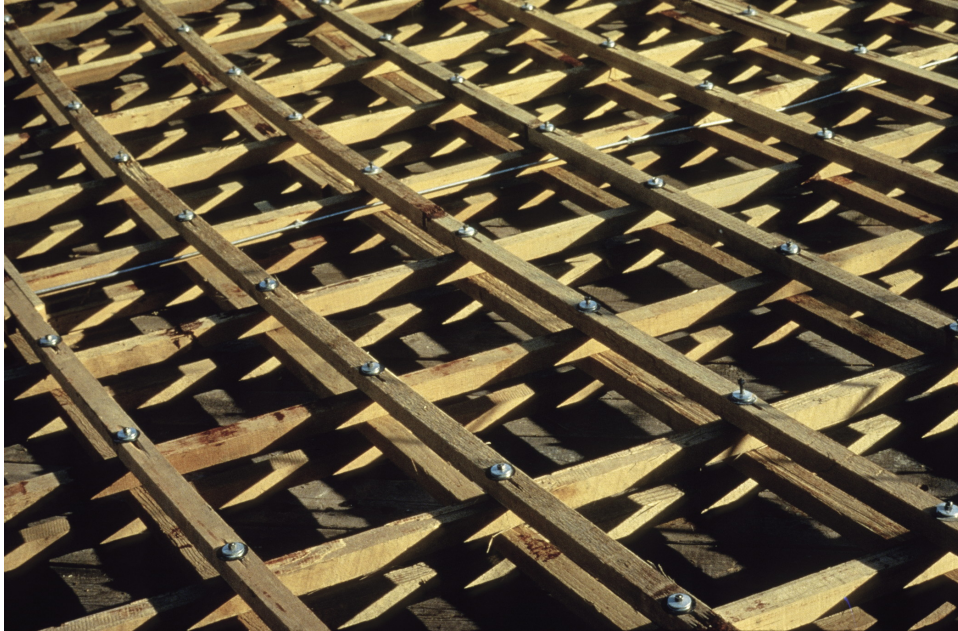
Figure 32: Mannheim gridshell 1974 by Mutschler & Partners, Freo Otto and Ove Arup & Partners - detail
