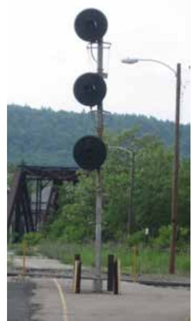
Figure 1: Northbound signal at the diamond crossing of the NECR and GMRC in Bellows Falls, VT dates from the 1960s and has reached the end of its useful life.
