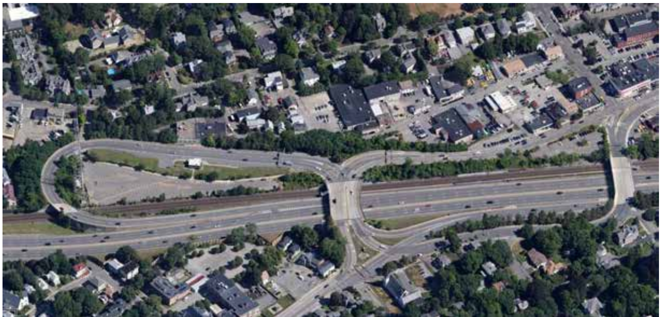
Picture 1: Aerial View of the Existing West Newton Station (Source: maps.google.com)
