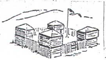
Fort Sullivan at Tioga
