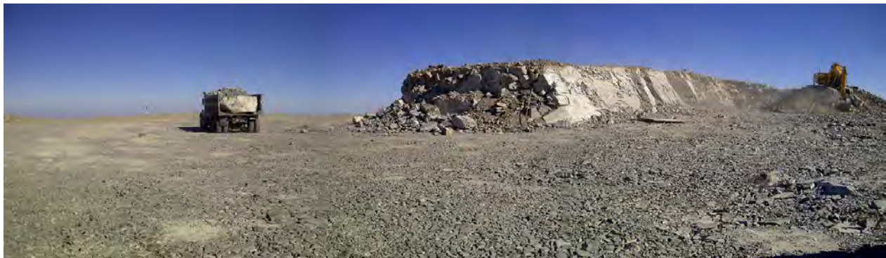
Figure 13 Clearing the GMT site. May 2012.
