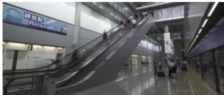
Current look of the West Hall APM platform, where two escalators are to be built to enhance the vertical flow of arriving passengers. 為改善抵港旅客的縱向人流，西大堂旅客捷運系統月台將興建兩部電動扶梯。圖為月台現時的面貌。
