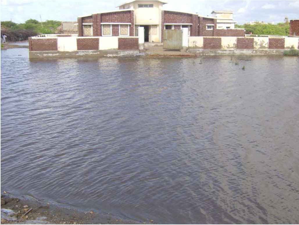
Plate 3: Inundation caused by 2003-Flood
