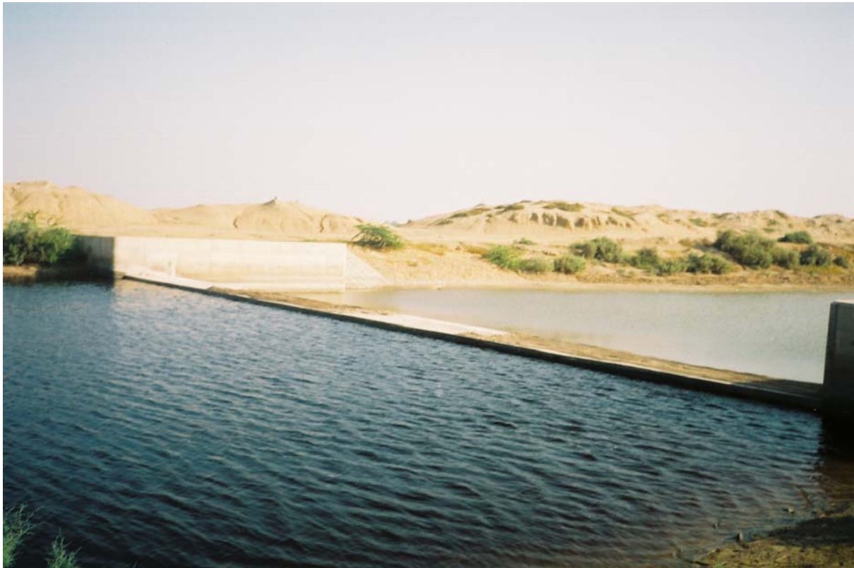
Plate 9: View of Weir at Head of DPOD looking Downstream (Nov. 08, 2007)
