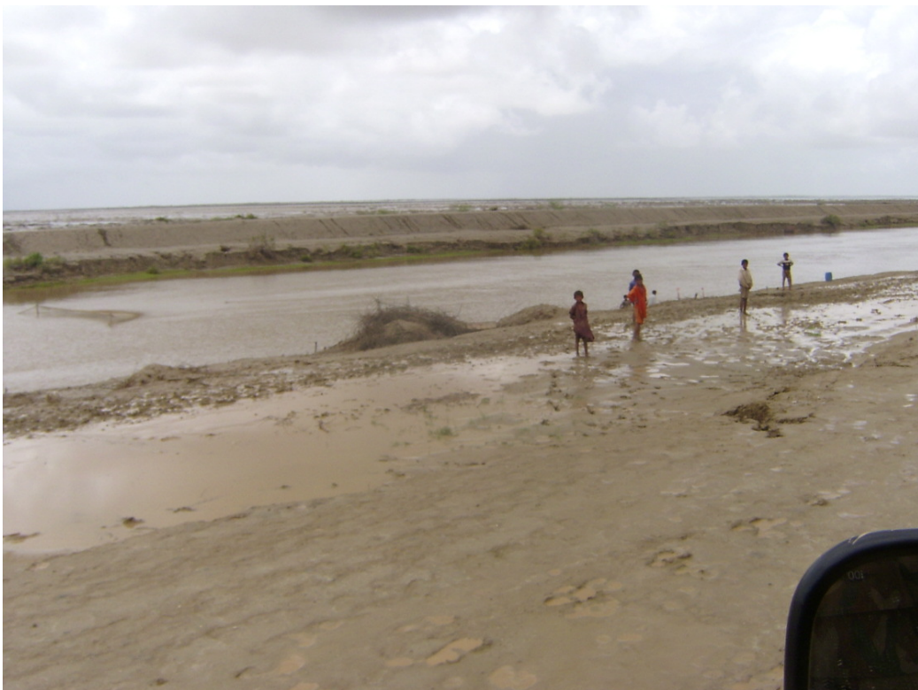
Plate 2: View of Berm of KPOD after Receding of Water of 2003-Flood
