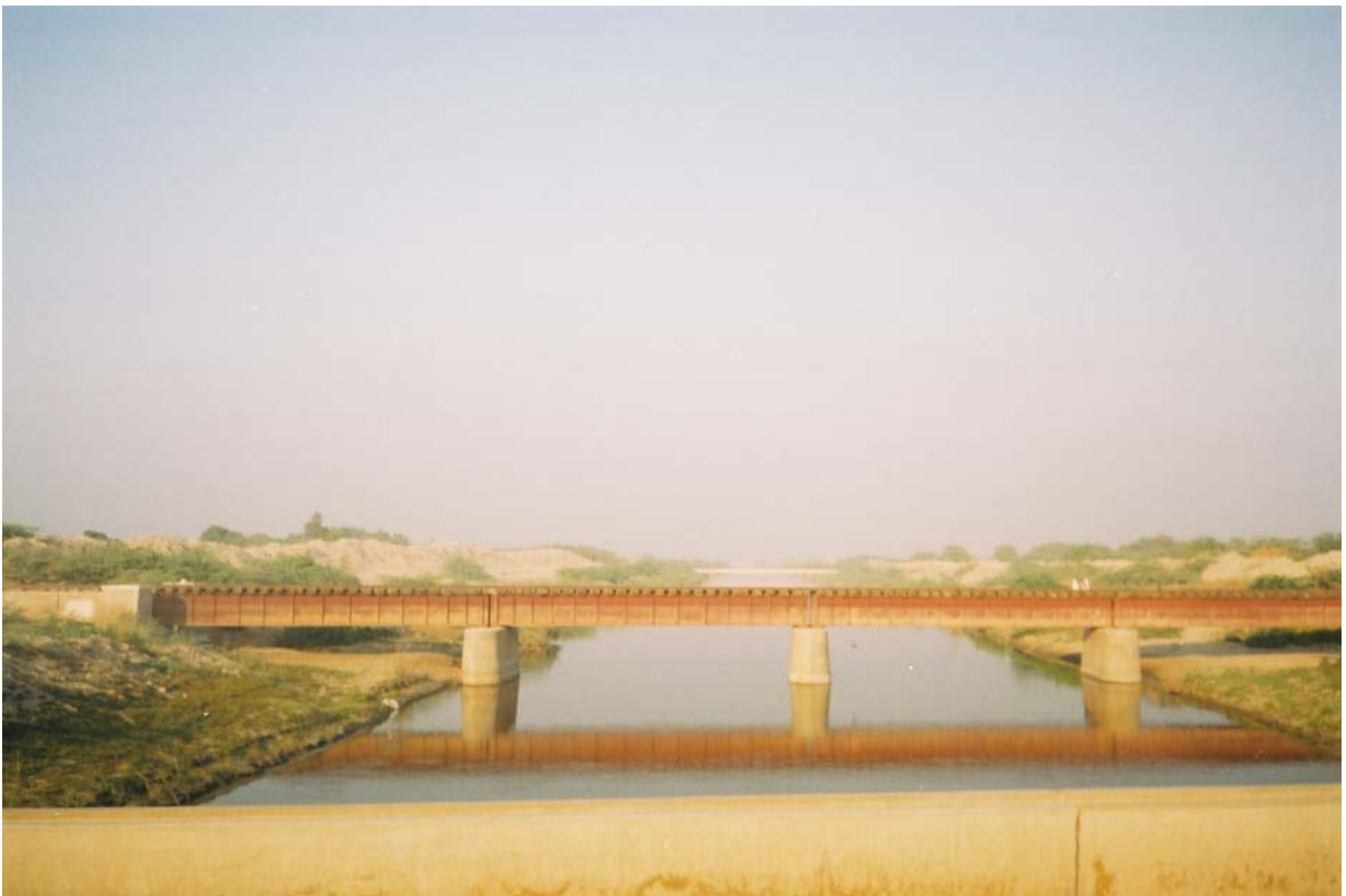
Plate 8: View of LBOD Upstream of RD 305 (Nov. 08, 2007)
