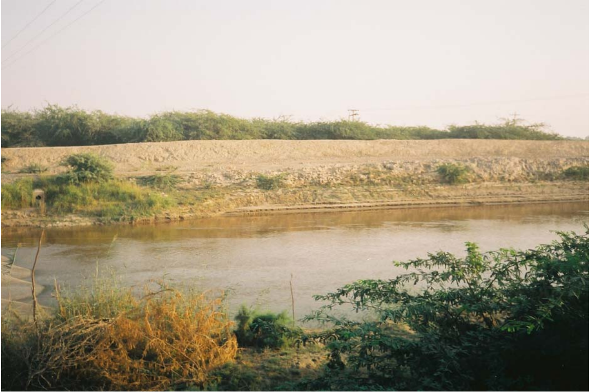
Plate 7: View of LBOD Downstream of RD 305 (Nov. 08, 2007)
