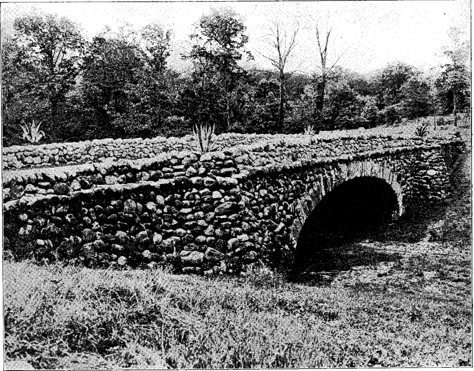
THE ZARTMANN BRIDGE, HIGHLAND PARK.
