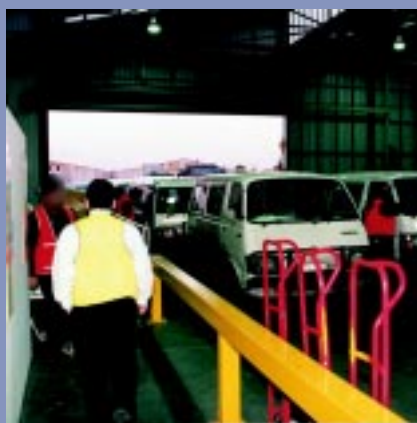
Figure 7.3 A good barrier system for separation of pedestrians from vehicle traffic.
