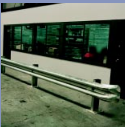
Figure 7.2 An 'Armco' barrier used to separate offices and pedestrians from vehicle traffic.
