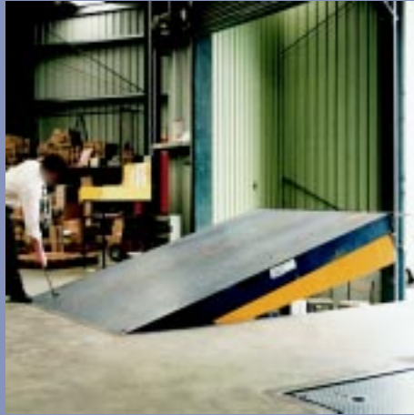
Figure 8.5 A well-designed levelling dock, illustrating the extreme range of its adjustment (Note: ramps should not be used at this angle).
