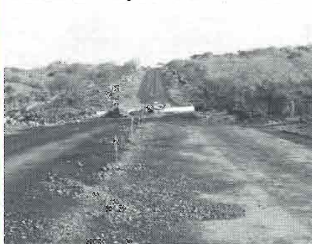
Excavation and subgrade continued in Kona.
