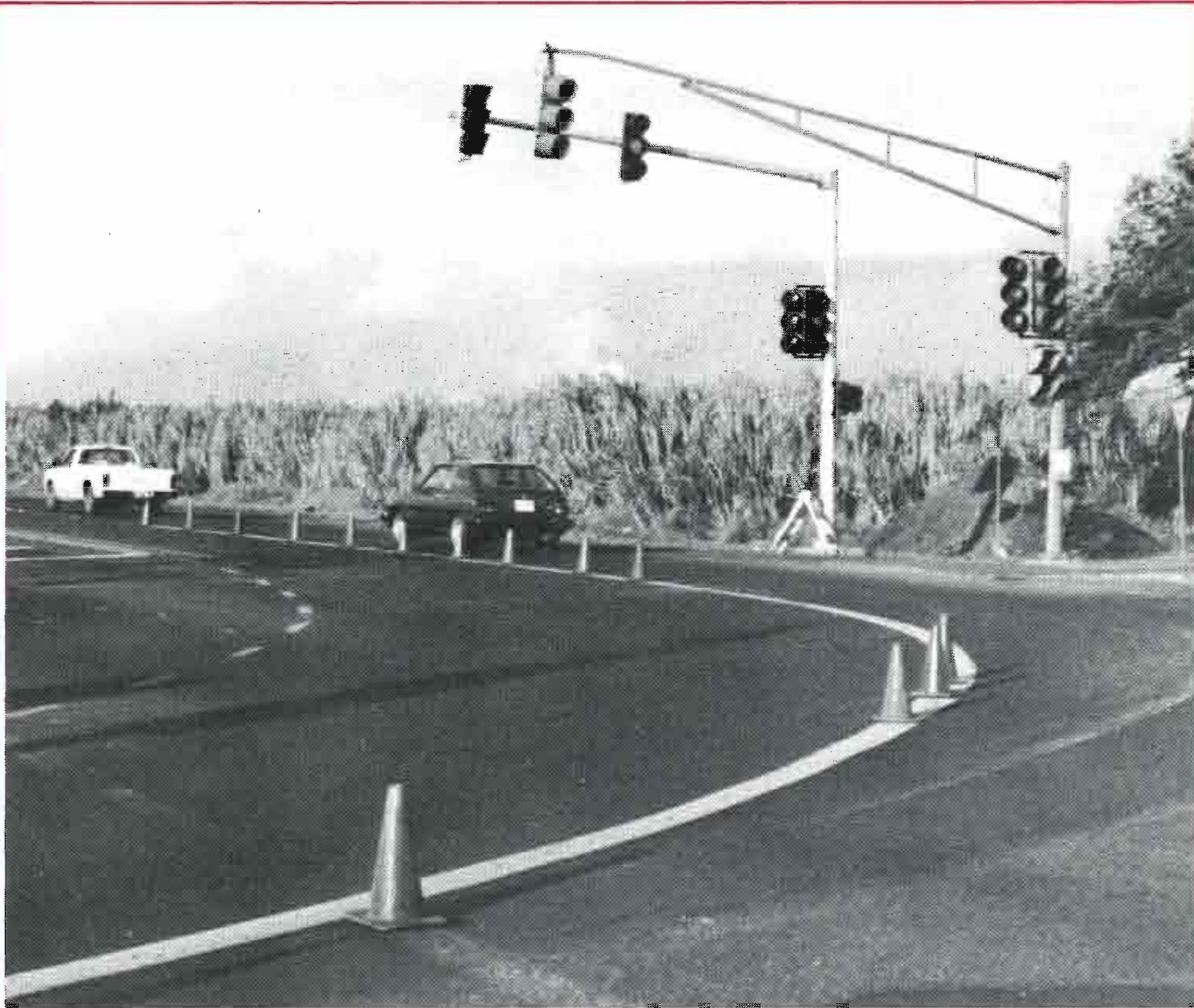
A new traffic signal on Hana Highway.
