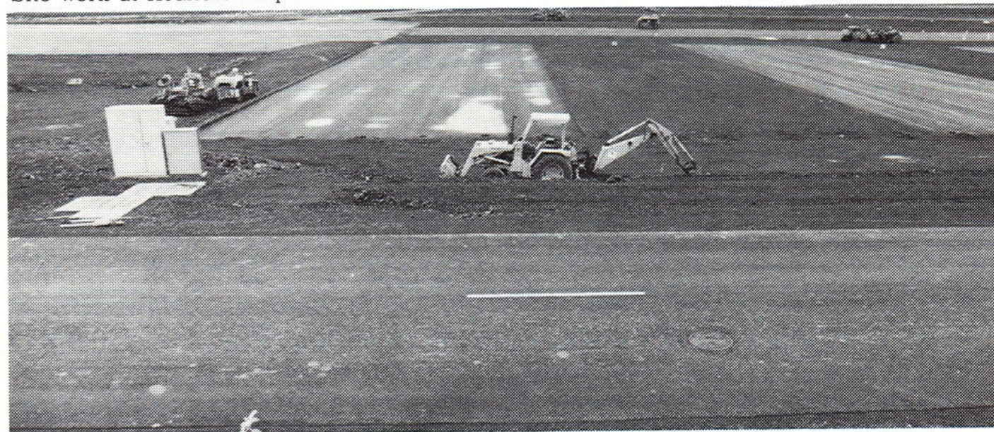
Site work at Keahole Airport
