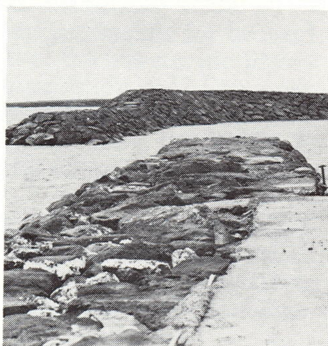
Breakwater at Port Allen Small Boat Harbor
