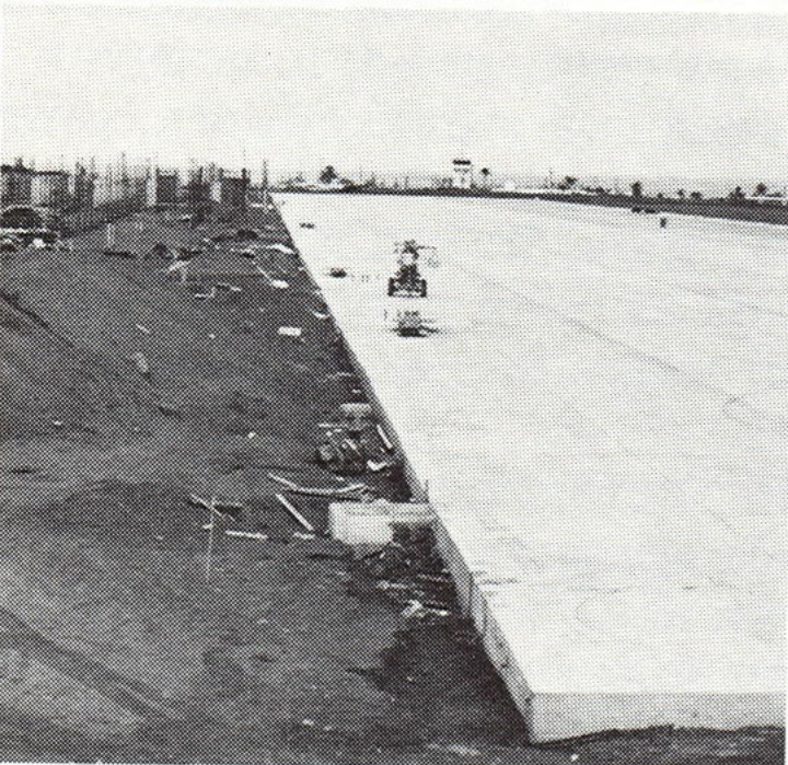
Site work at Lihue Airport
