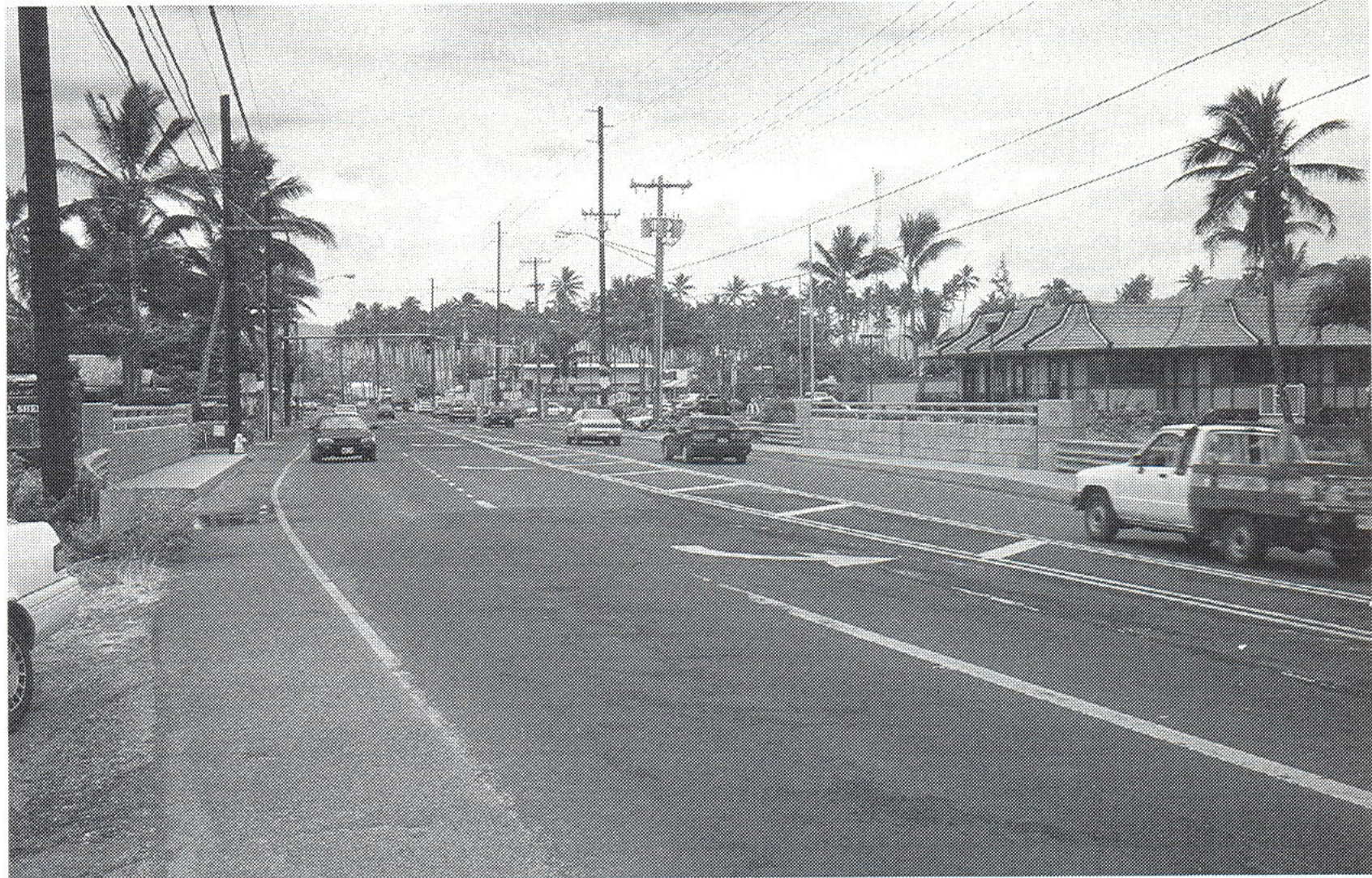
Efforts to relieve traffic congestion on Kauai included widening and adding a left turn lane to Uhelekawawa Bridge.
