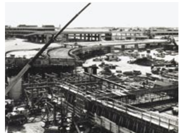
Top: Construction on the Central Concourse. Above: Elevated roadway construction.
