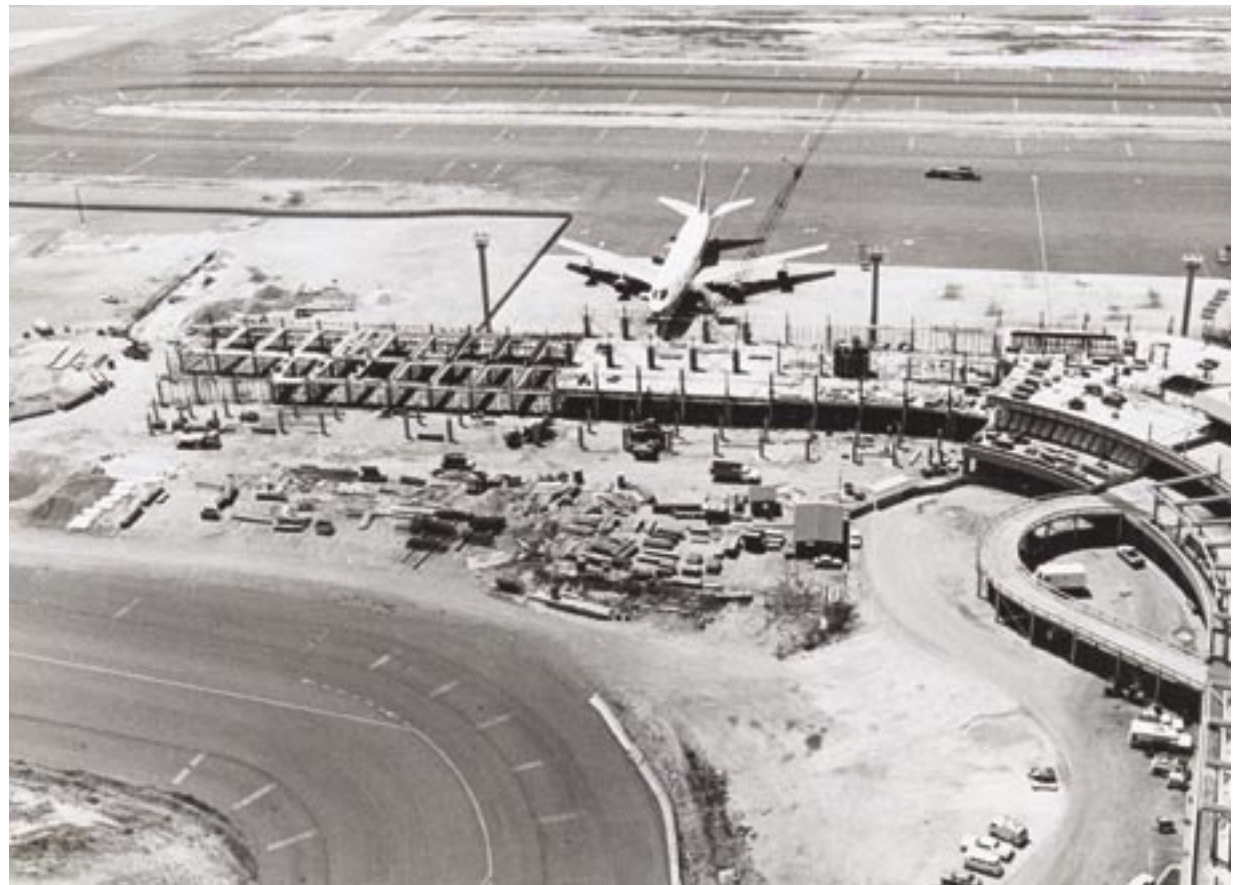
Below: Aircraft park amid construction activity on the Diamond Head Concourse.
