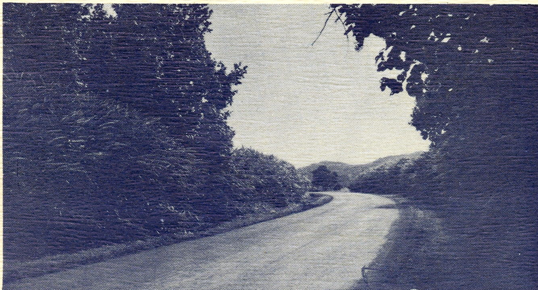
KAUAI BELT ROAD—Typical Maintenance.
