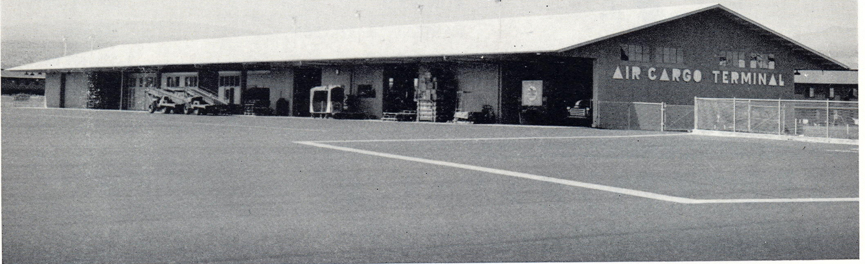
New air cargo terminal building at General Lyman Field.
