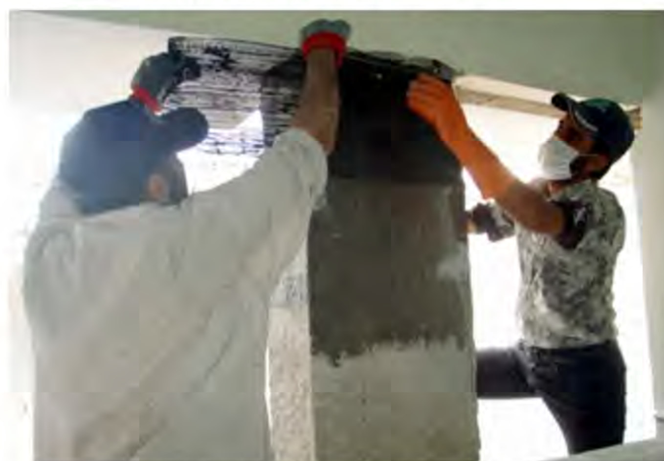
Retrofitting of Jinnah Dental Hospital Building Muzaffarabad
