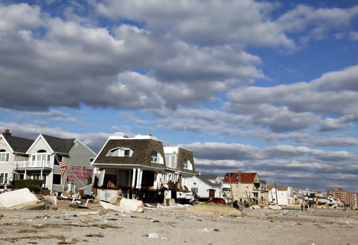
Destroyed beach houses in the aftermath of Hurricane Sandy, November 4, 2012 in Far Rockaway, NY.
