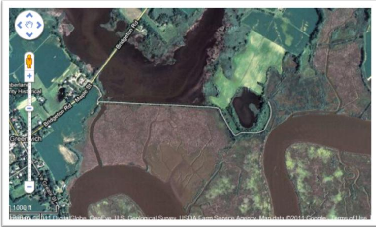
Photo 5: Pine Mount - Mill Creek dike provides flood protection and protects freshwater resources. Image: Google
