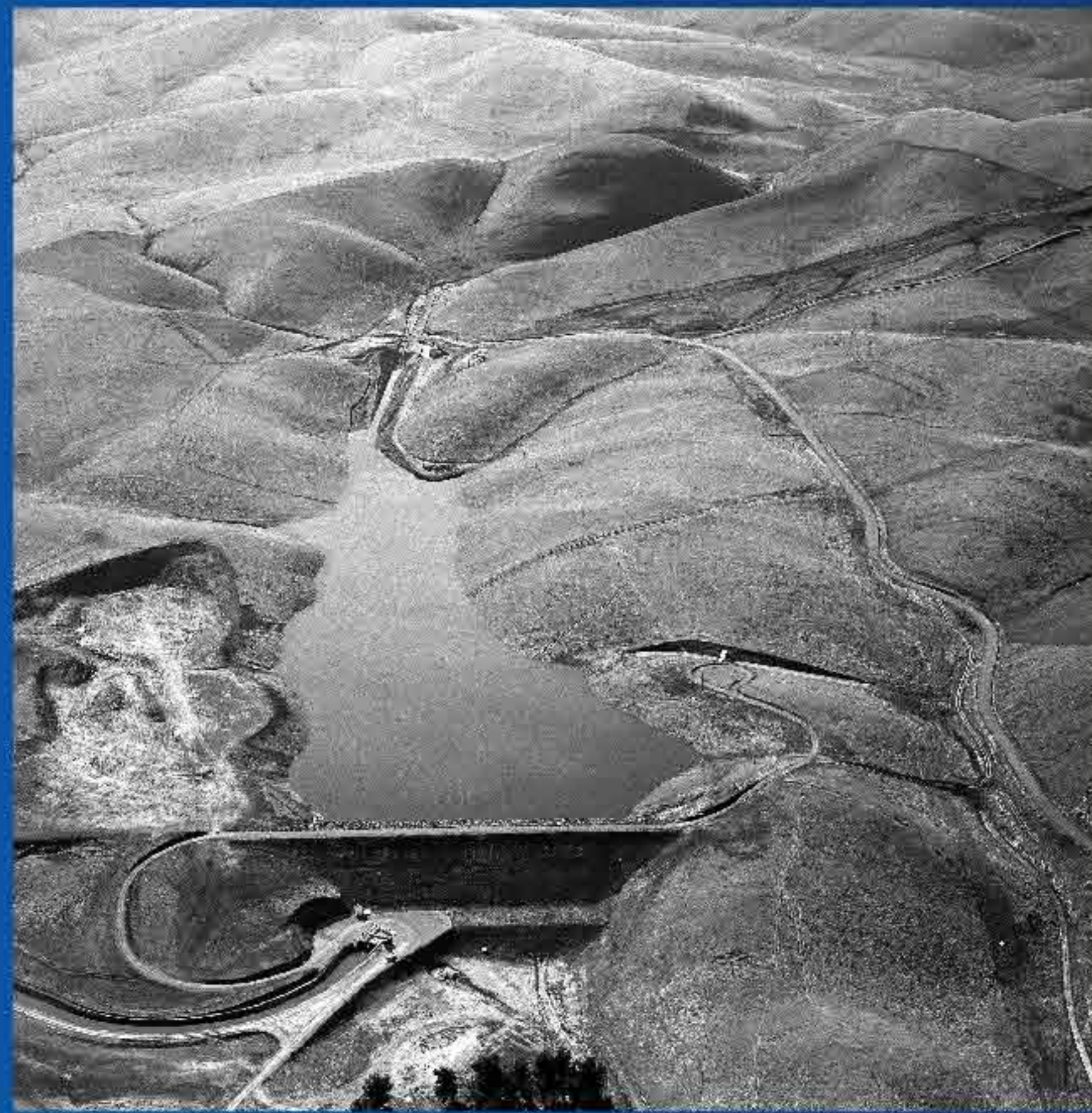
1960 photo showing South Bay Pumping Plant with Bethany Dam and Forebay in the foreground.
