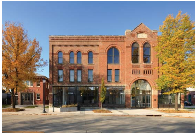
Hose Station No. 4 and C.S.P.S. Hall (photo: Emily Myer)
