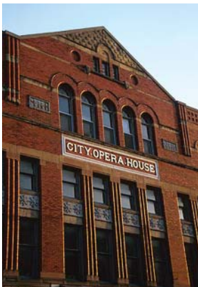
The City Opera House, (photo: NPS project file)
