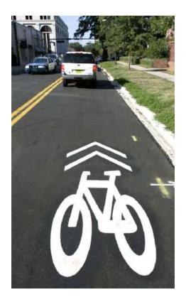
FIGURE 5 - "SHARROW" PAVEMENT MARKING (Source: National Committee on Uniform Traffic Control Devices 2007)
