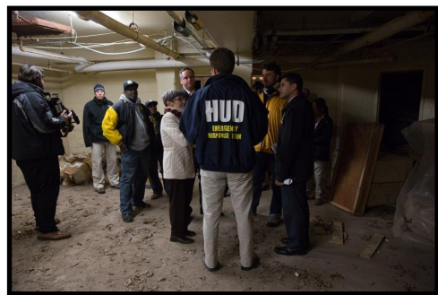
HUD’s Emergency Response Team inspects Hurricane Sandy damage.
