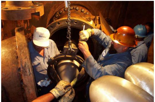
Installation of prototype nozzle seat ring and needle tip Figure 5
