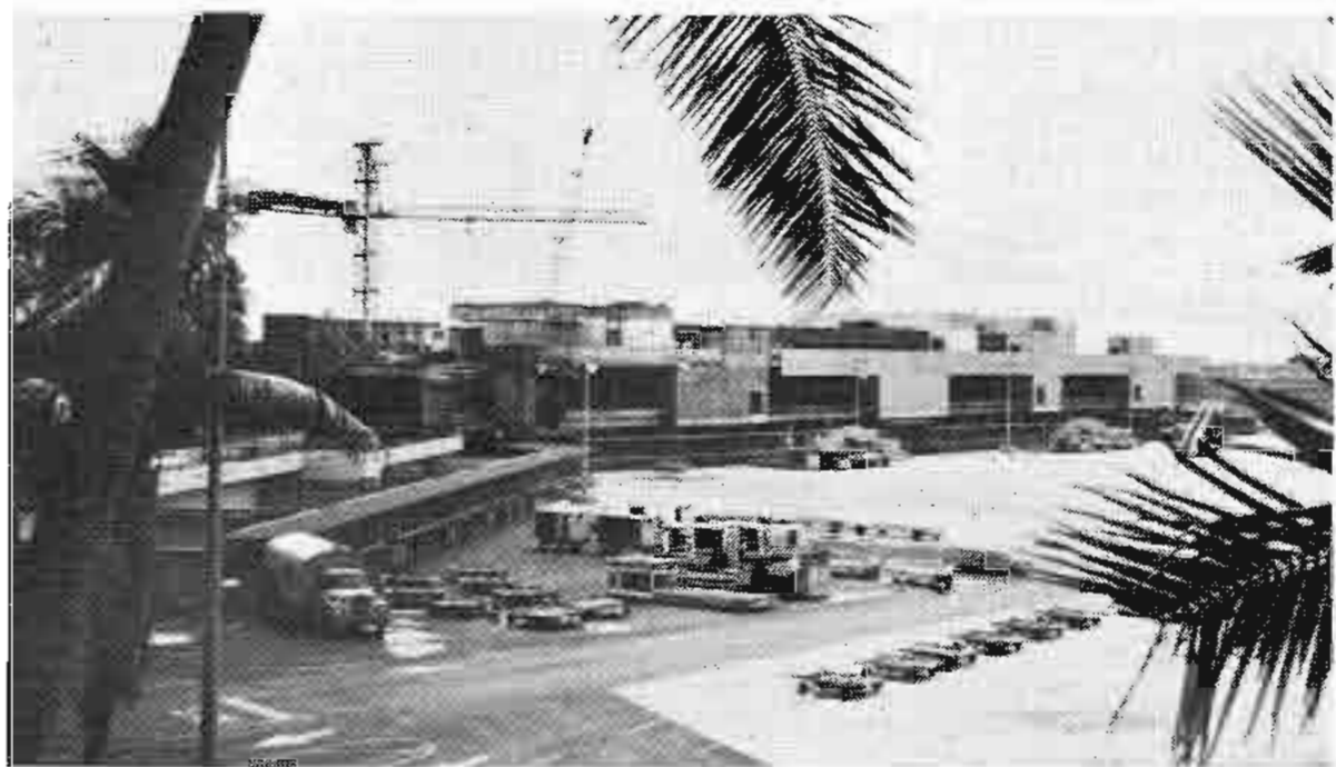
Construction of Central Concourse at Honolulu International Airport.
