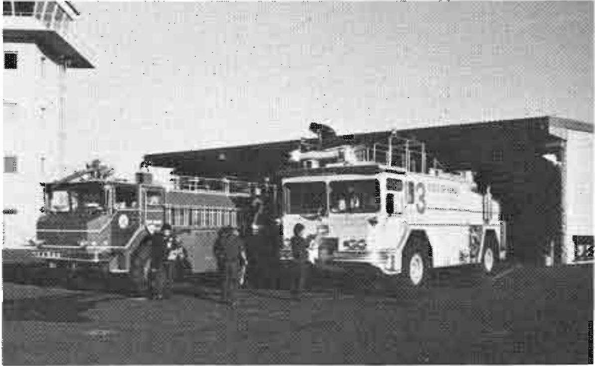
New Crash-Fire Station at Lihue Airport.
