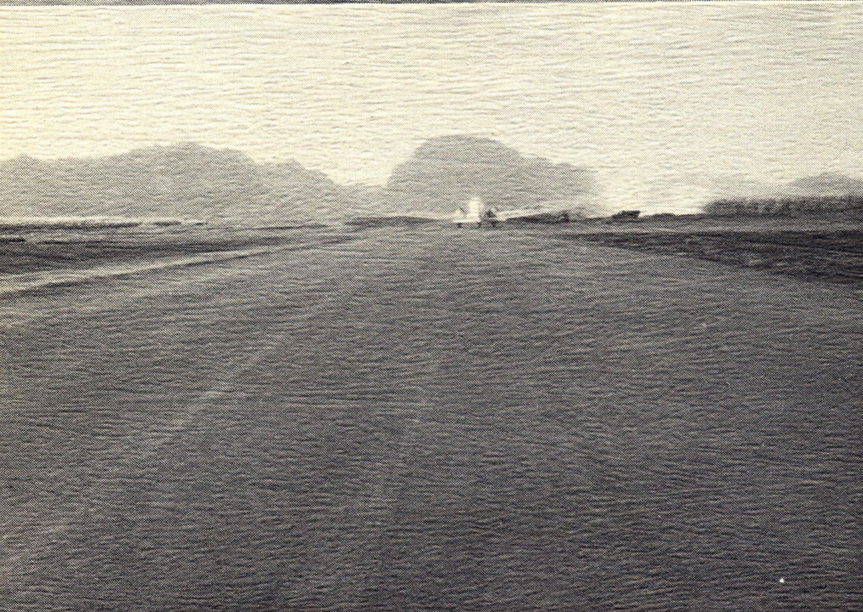
Lihue Airport. Contract involving construction of additional paved areas. Above, completed auto park. Bottom, completed parking apron.
