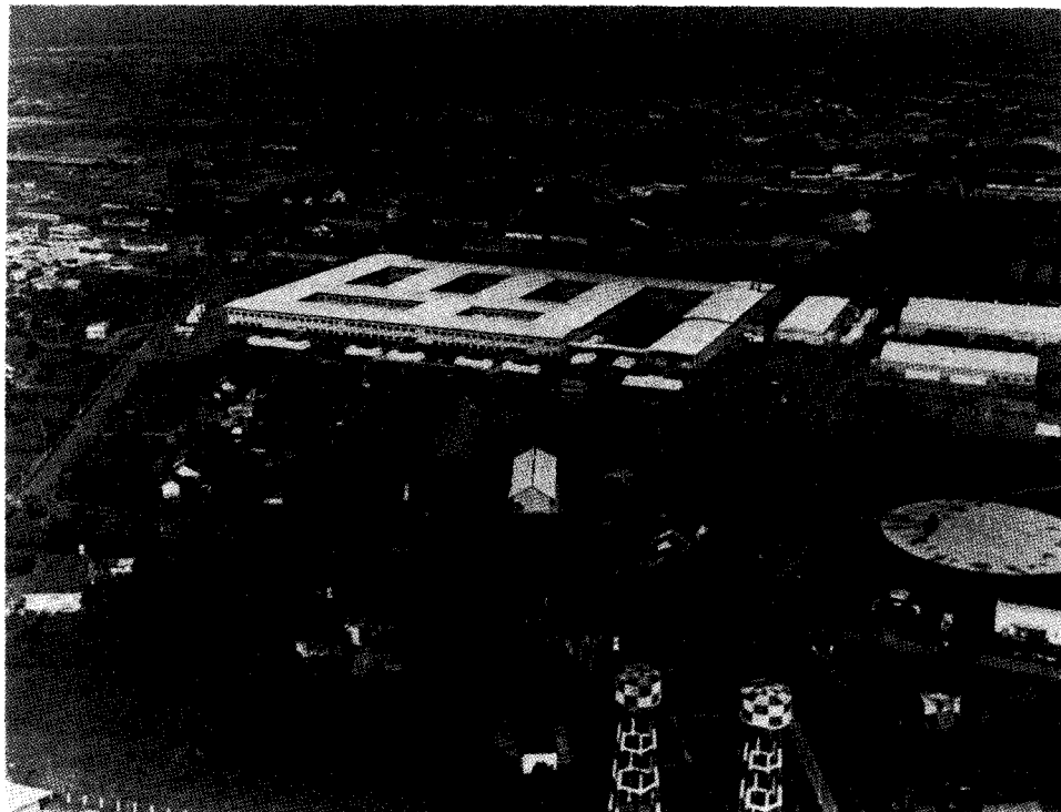
MACV Headquarters, with Tan Son Nhut Air Base in the background
