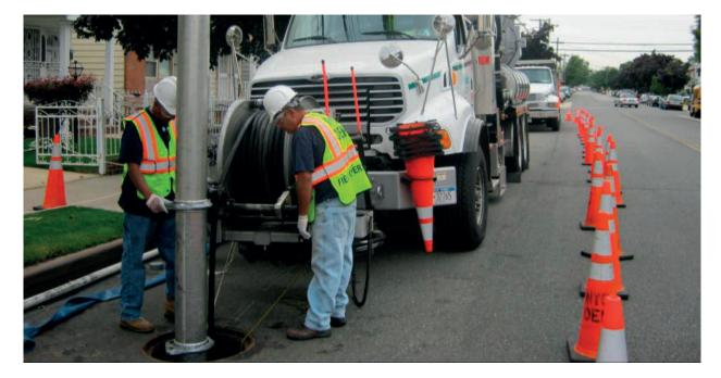
Figure 13: DEP Crew and Vactor Truck in Operation
