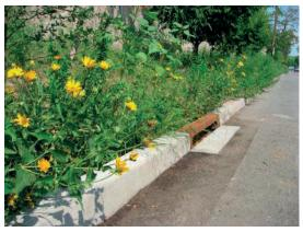
Low Density Residential Street: Post-Construction Infiltration Swale
