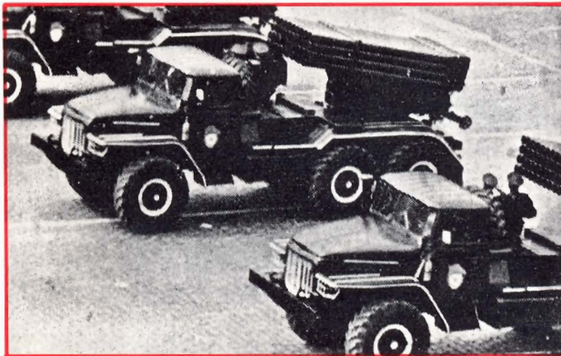
A series of free rocket over ground [FROG] missiles and their carriers are in the Russian Army inventory. Pictures here show a BM-21 standard artillery rocket launcher of the Warsaw Pact armies that is widely exported. The 122-mm rockets are fired from 40 cell launchers mounted on a URAL-375 6 by 6 truck. Czechoslovakia has the launcher mounted on a Tatia 813 8 by 8 vehicle with reload carried.
