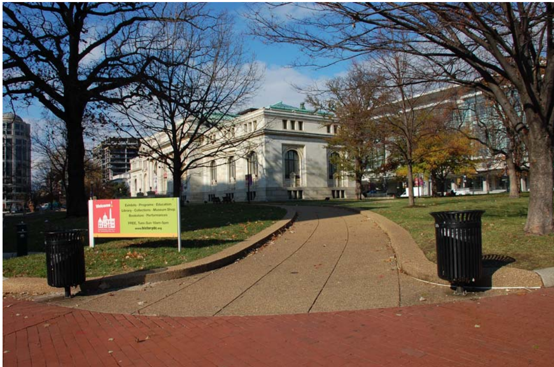
Figure 2 - View west to the Carnegie Library building at Mount Vernon Square
