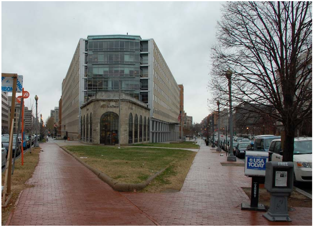
Figure 2 – View west to Reservation 78
