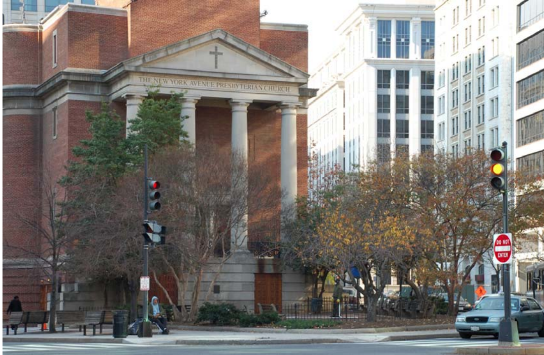
Figure 1 – View west to Reservation 172
