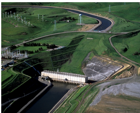
Harvey O. Banks Pumping Plant.
