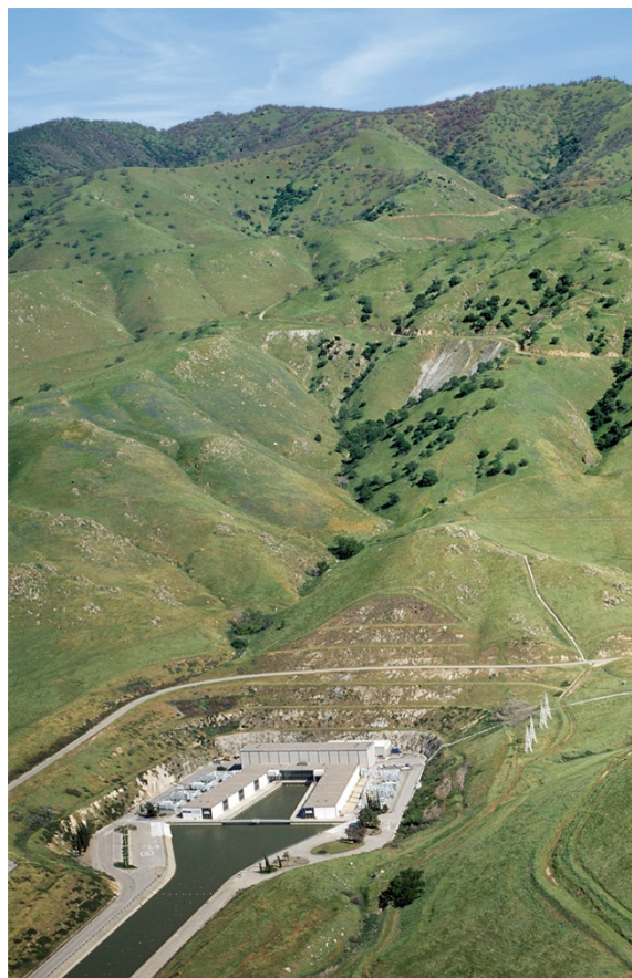
A. D. Edmonston Pumping Plant.
