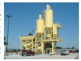
There are two main types of concrete batch plants: truck mix and central mix. Truck mix batch plants load out the ingredients of the concrete mixture into a mixer truck, and the truck mixes them to form the concrete. Central mix facilities mix the ingredients internally before being loaded into the truck.
