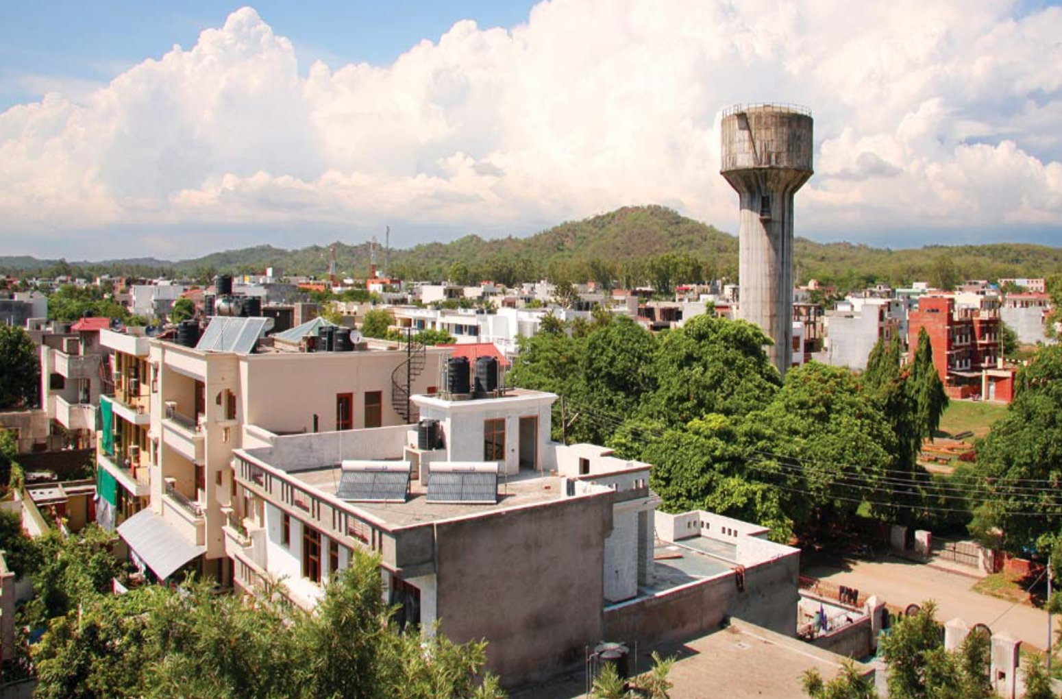
A housing complex: Nestled in the hills
