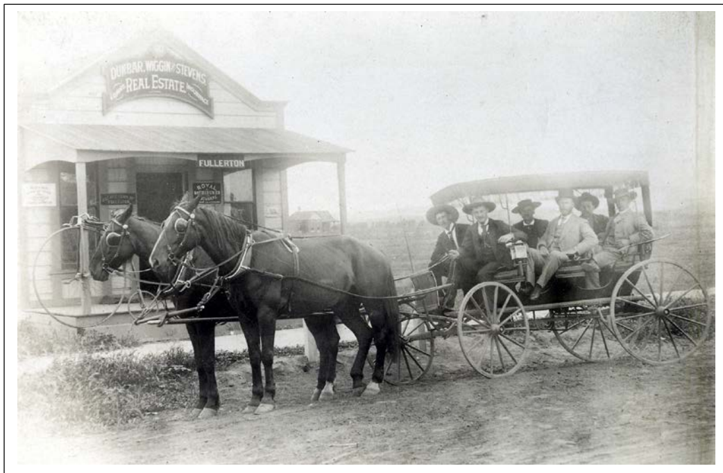
Image 9: Building located on the east side of Spadra Road (now Harbor Blvd.), ca late 1890s Source: Fullerton Public Library, Local History Room
