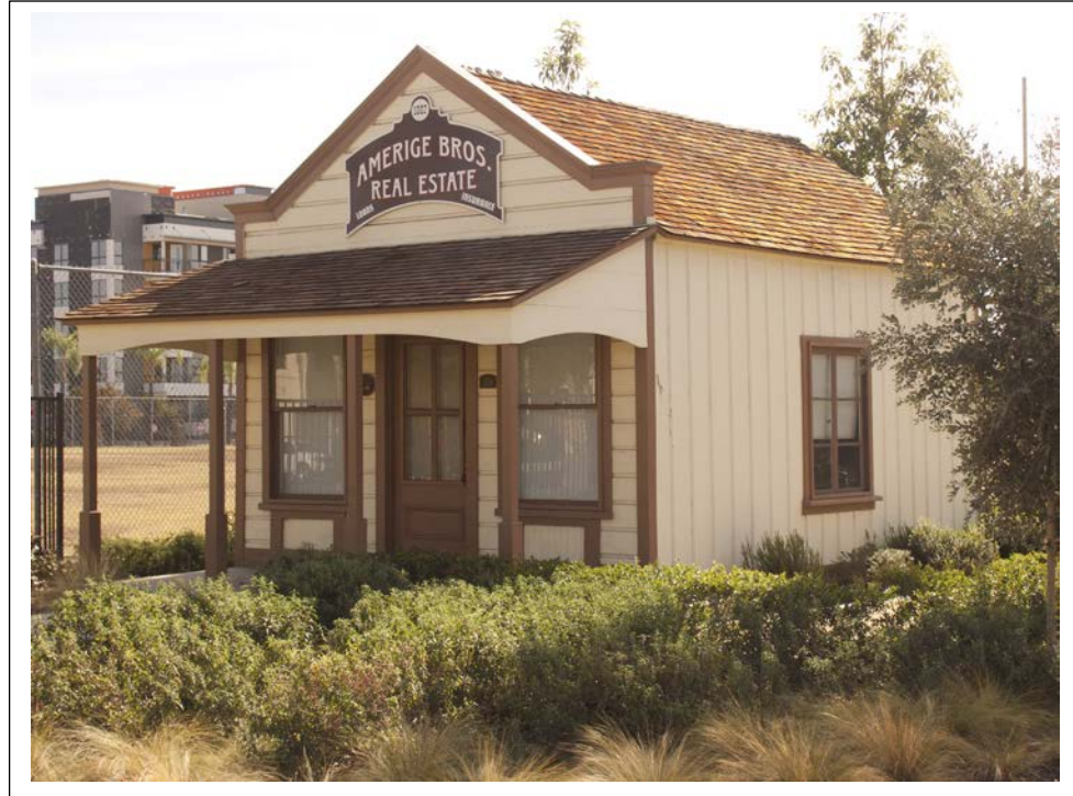
Photo 5: Front elevation, looking southeast
