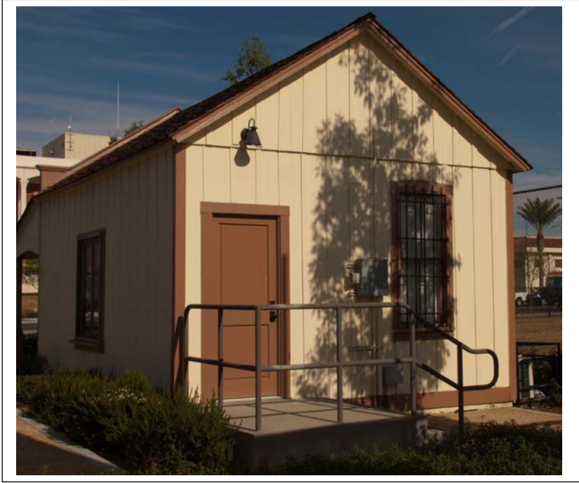
Photo 3: South (rear) elevation
