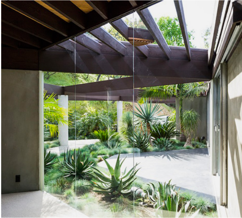
Detail of trellis (© The John Lautner Foundation, courtesy of Frank Escher, date of photograph unknown)
