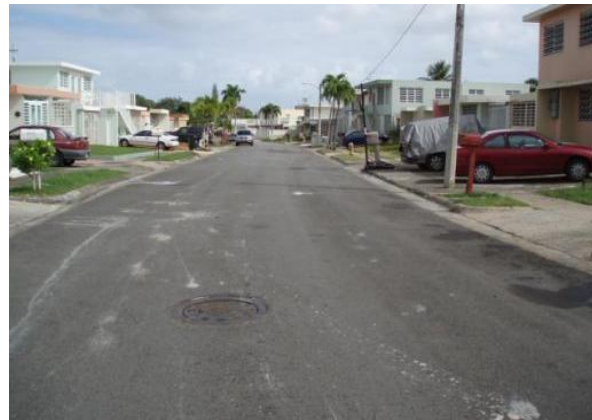
A typical Puerto Rico road right-of-way (ROW) includes travel/parking lanes, utilities, street trees, and sidewalks.
