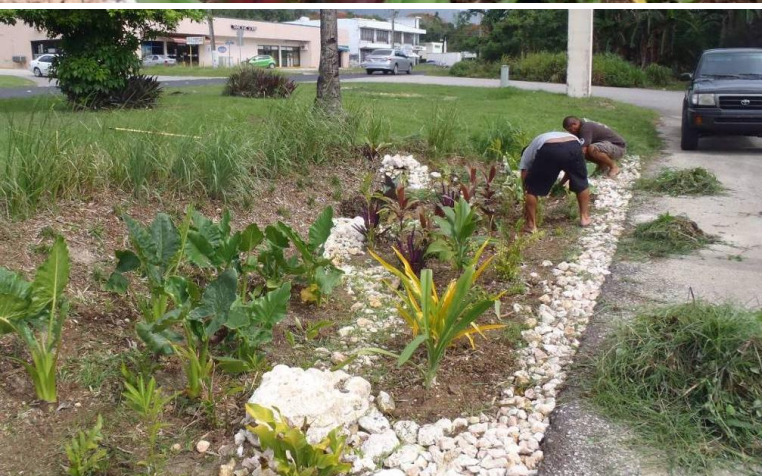
Maintenance activities for vegetated BMPs include: watering after installation until plants are fully established; and weeding, particularly during the first year.
