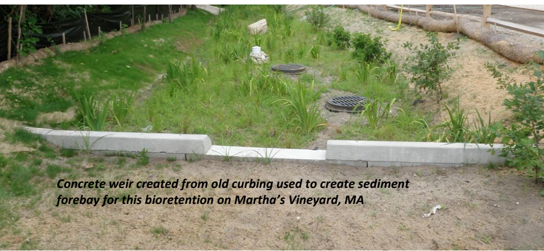
Wide grass filter strips as parking provide pretreatment.
