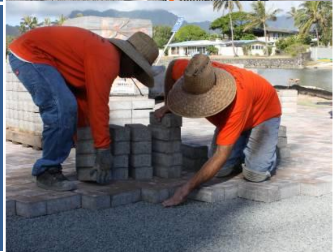
Pavers installed and leveled over bedding stone
