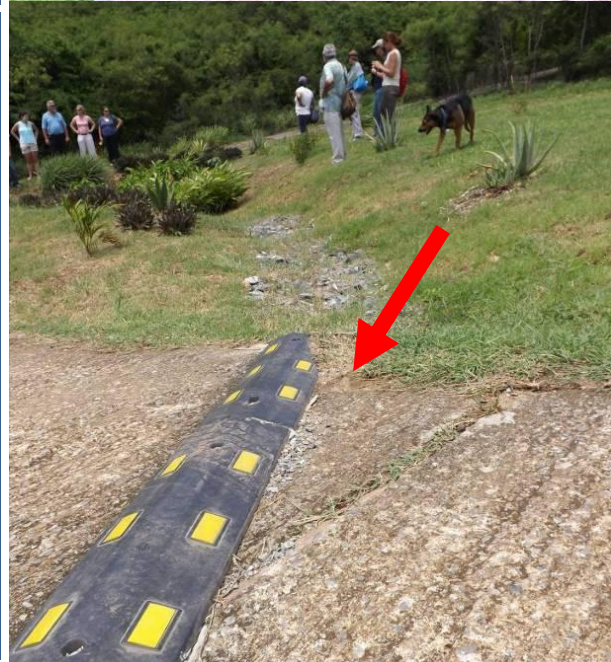
Arrow indicates sediment build-up at pavement/swale interface
