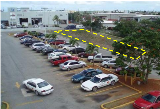
This retailer on Guam uses a ponding basin for temporary detention of parking lot runoff.
