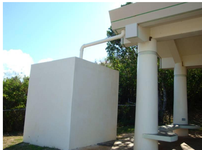
Islands have an inherent interest in rainwater harvesting to reduce the burden on drinking water supplies. Cisterns are commonly used for small-scale potable water or to satisfy non-potable needs (e.g., irrigation, toilet flushing, car washing, fire suppression).
