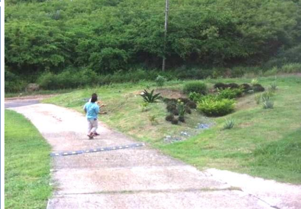
Completed Rain Garden – 7 months after construction
