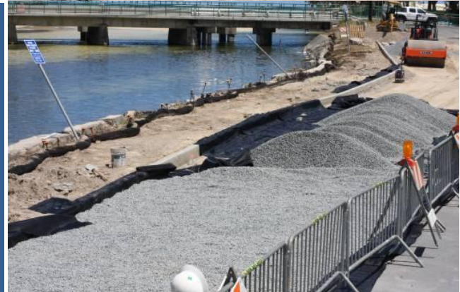
Stone sub-base with geotextile fabric separating the sub-grade
