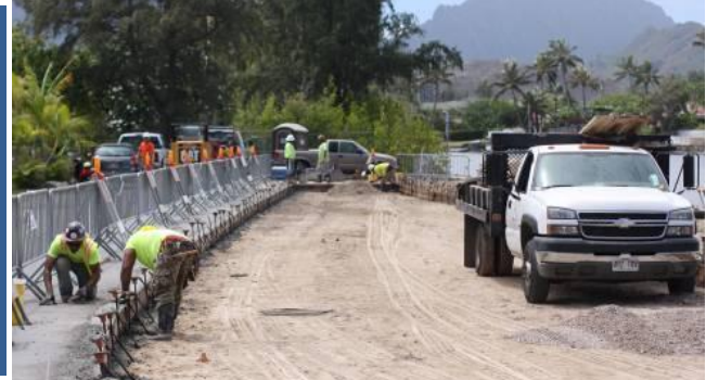
Removal of existing pavement surfacing
