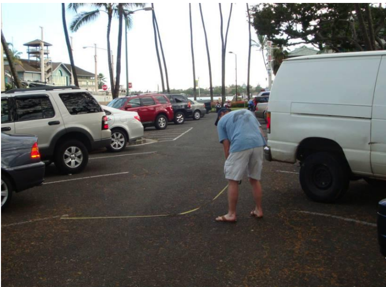
LID includes site design techniques to minimize the amount of impervious cover used on a site, like this parking lot in Honolulu that uses narrow drive aisles and small parking stalls.
