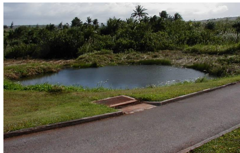
Ponding basins for infiltration (top) and wet ponds that maintain a permanent pool (bottom) can often be improved to increase treatment performance.
