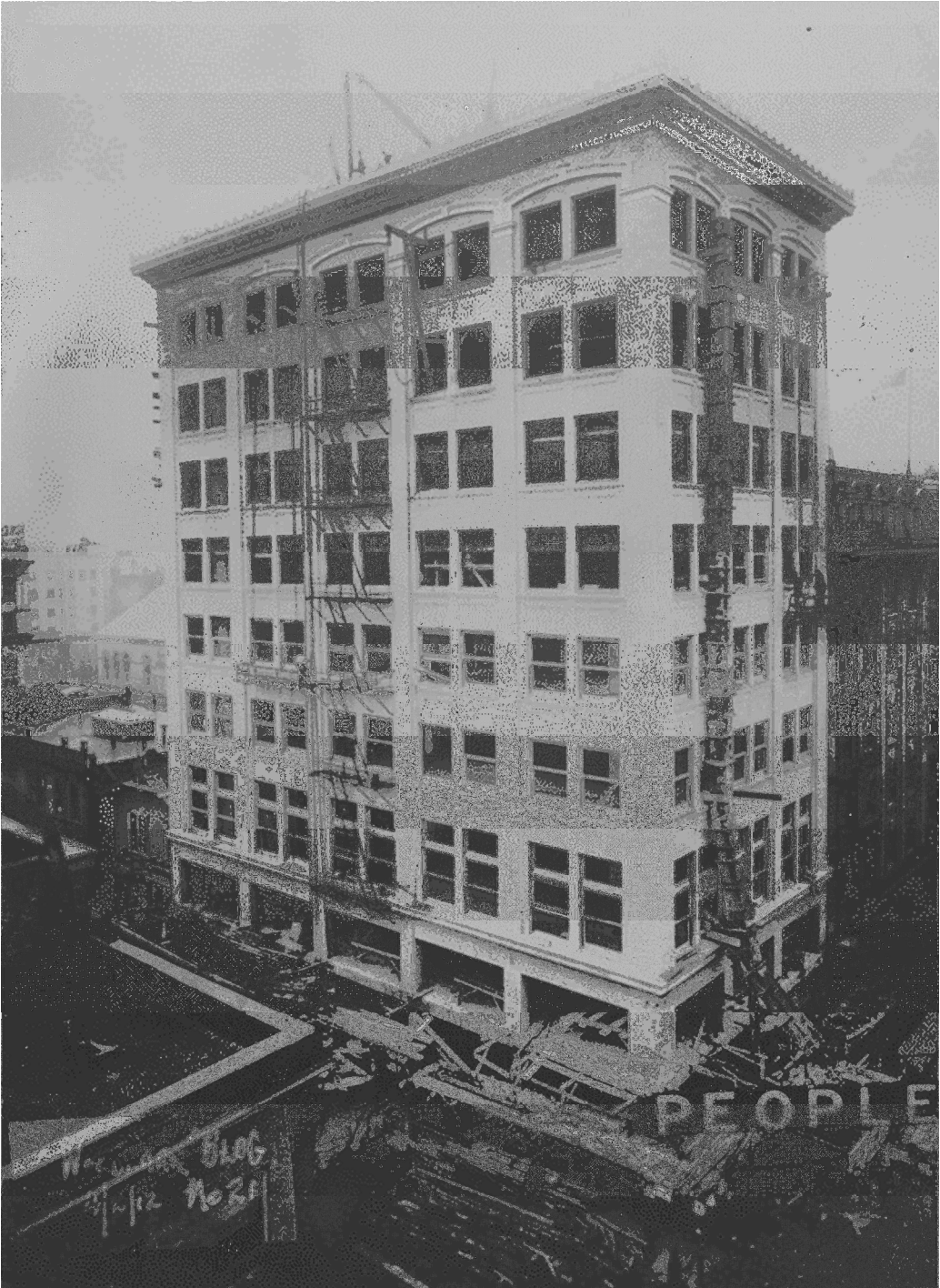
FIGURE 7: Woodlark Building Construction, April 2, 1912 (OHS bb011290)
