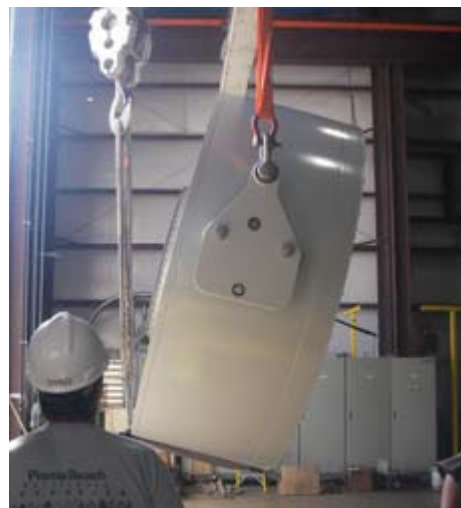
Figure 4-10. The generator was rotated into position using a three-point lift, to be as safe as possible.
