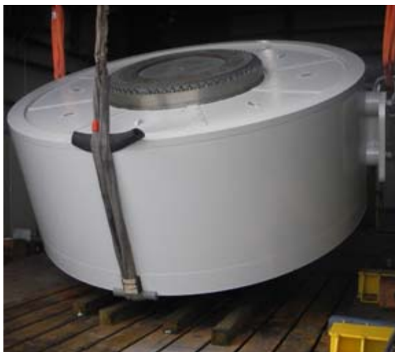
Figure 4-10. The generator was rotated into position using a three-point lift, to be as safe as possible.
