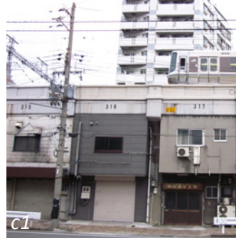
(c) (infra)structural gaps
