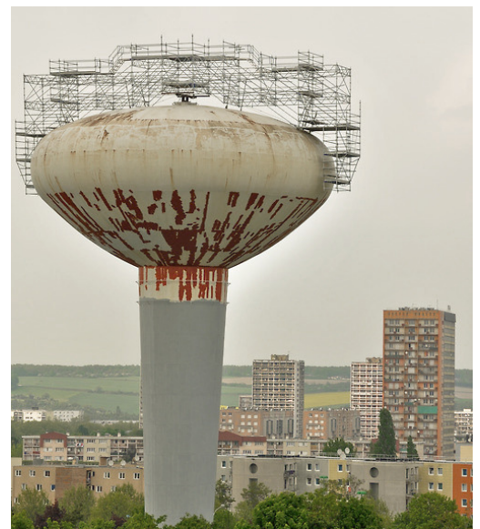
Figure 5.14 Scaffolding conforming to unique form
