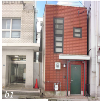
(b) gaps between buildings
