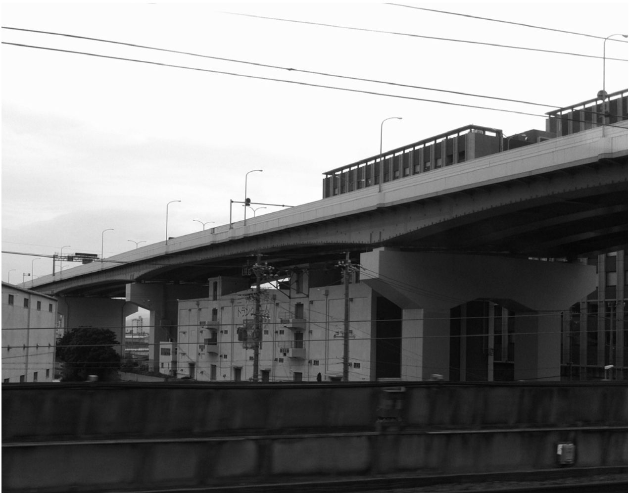
Figure 2.6 Modern ambivalence: Elevated highway built over an existing warehouse in Nagoya
