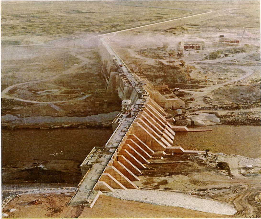
Fig3.3: Aerial view from the east bank
