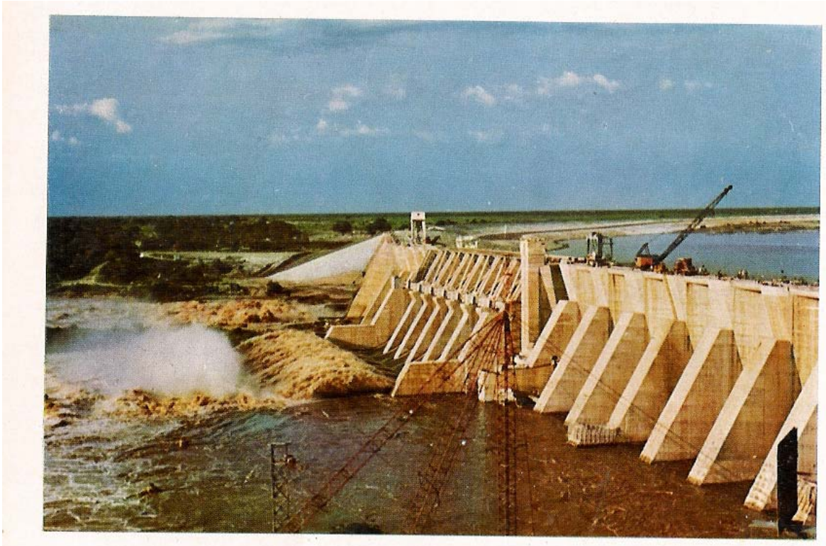
Fig 3.2: Passing flood water in Roseires dam
