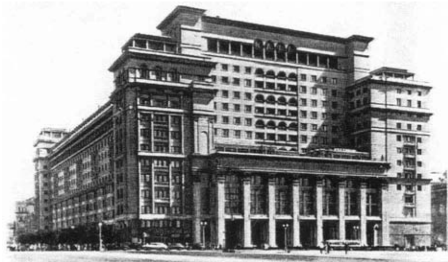
91. Alexej Stschusev, Leonid Saveljev, Osvald Stapran. Mossovet-Hotel in Moskau, 1933.
