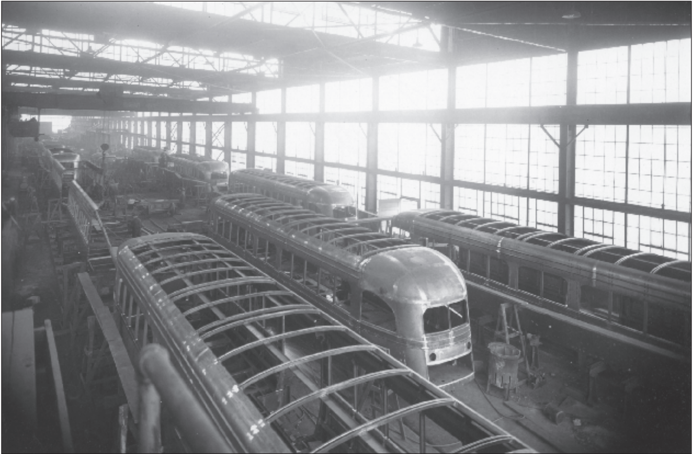
The fabrication of PCC bodies is in full swing at the St. Louis Car Company's erecting shop circa 1938. Washington University in St. Louis, Special Collections - St. Louis Car Co.
