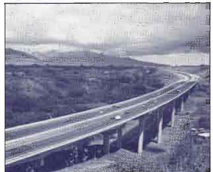
The Kipapa Bridge on the H-2 Freeway was completed in 1977. It is the highest bridge on Oahu (156-feet) and was the first cantilivered, cast-in-place, segmental bridge in Hawaii.
