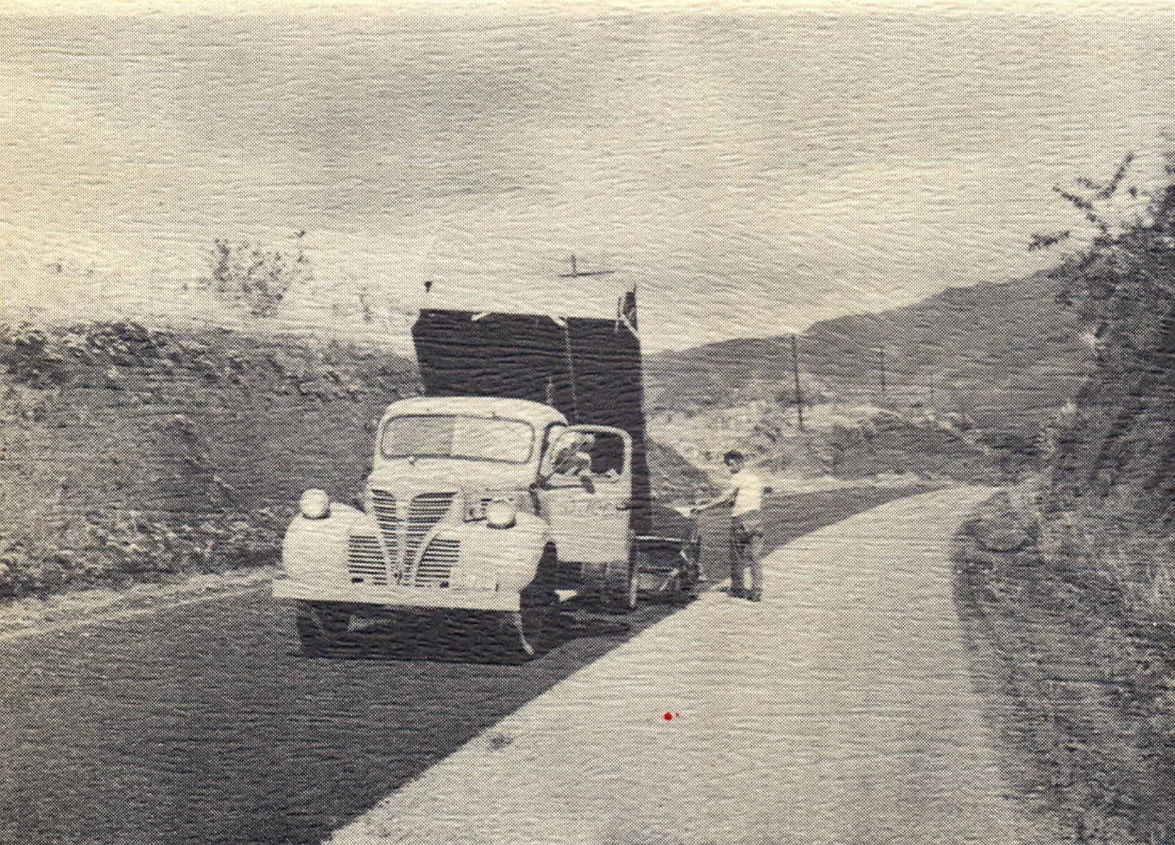
Resurfacing and widening Kauai Belt Road between Koloa junction and Lihue.
