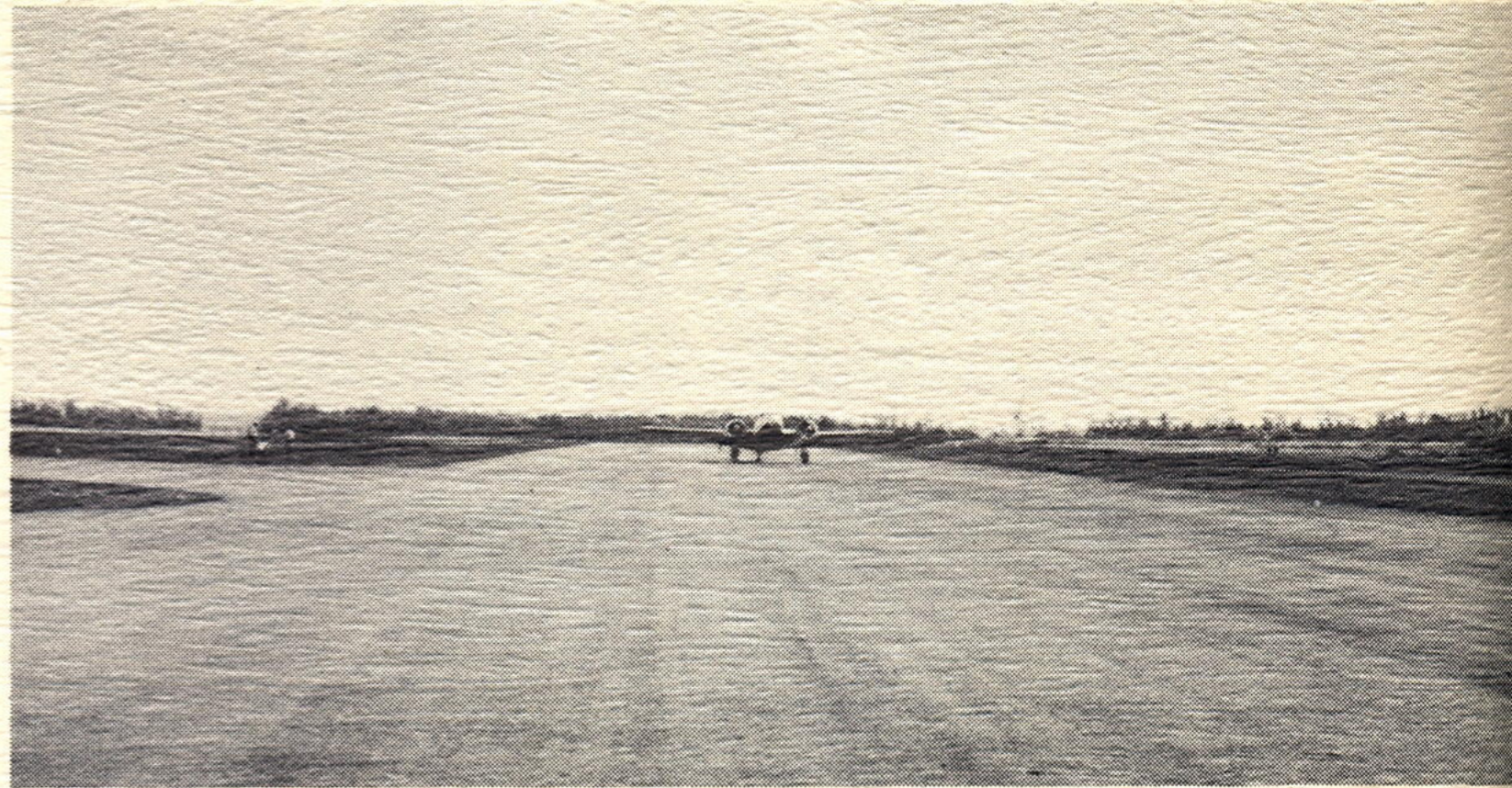
Completed runway, Lihue Airport. Runway is 3,750 feet long. Project's cost including parking apron was $384,395.
