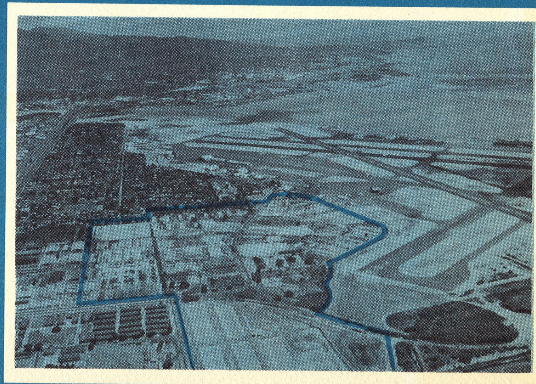
Old NAF area as cleared for airport expansion.
