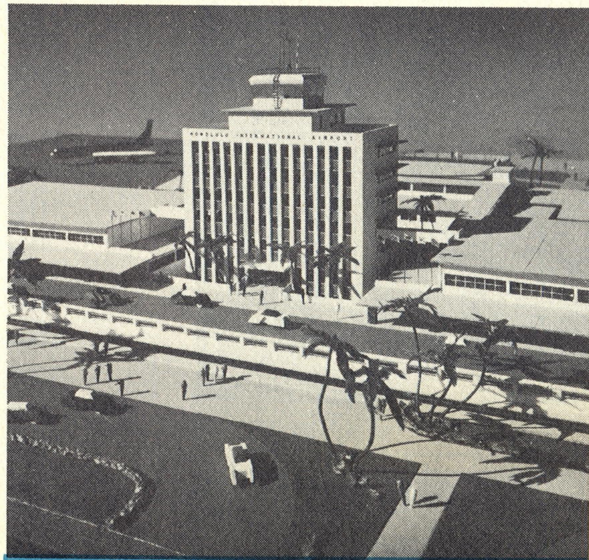
Passenger unloading from street ramp at second floor level.
