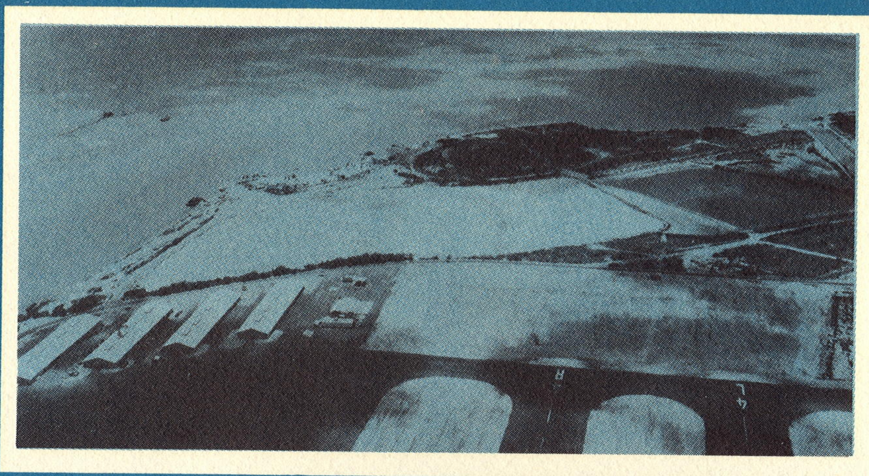
Coral fill stock pile area, Honolulu International Airport.
