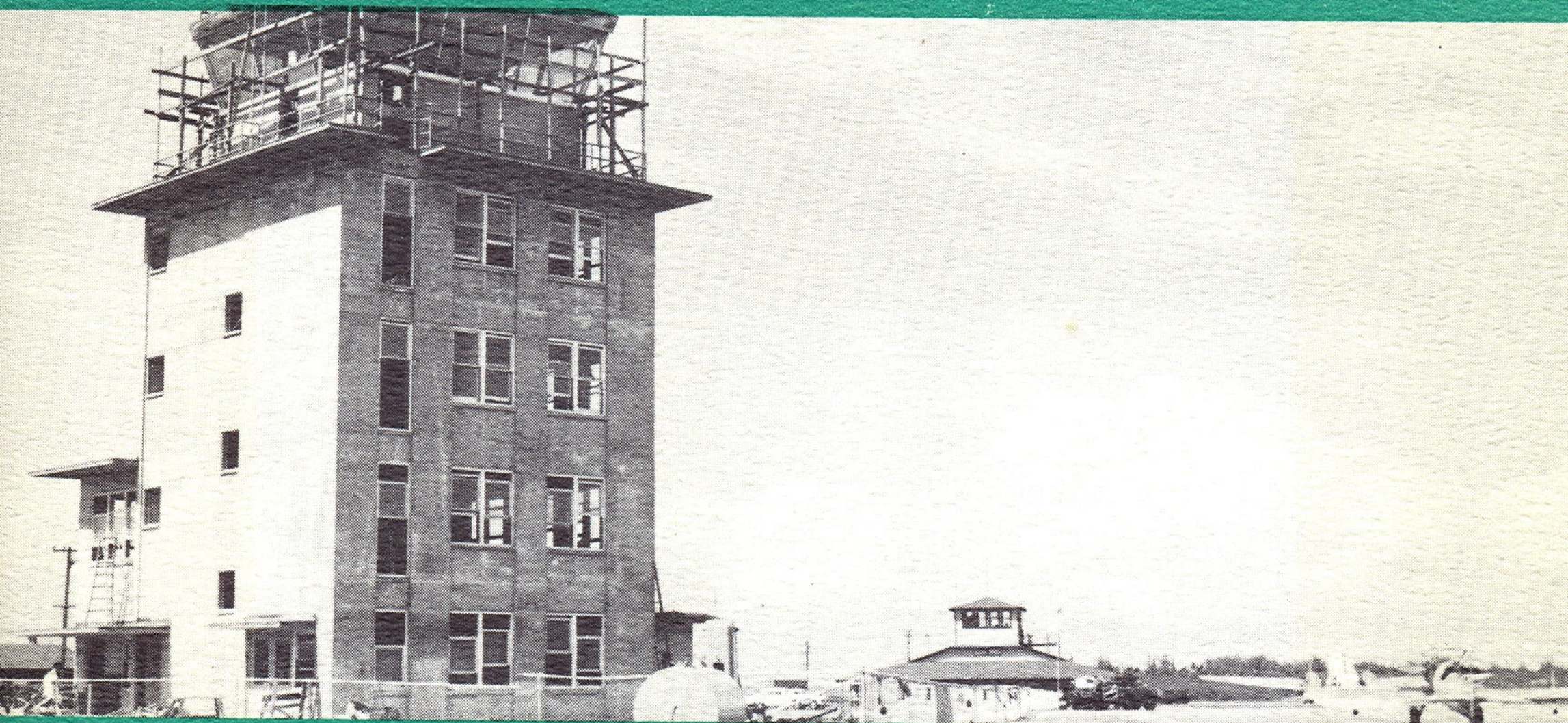
Kabului Airport. New tower under construction in foreground.
