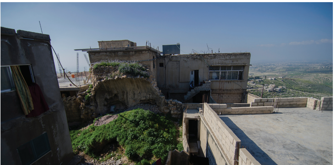
View of one of the villages in Irbid, Jordan. NRC estimates that across Irbid, Jerash and Ajloun governorates the Urban Shelter Programme has already met the shelter needs of 8% of the registered Syrian refugee population. ©Alisa Reznick, March 2015
