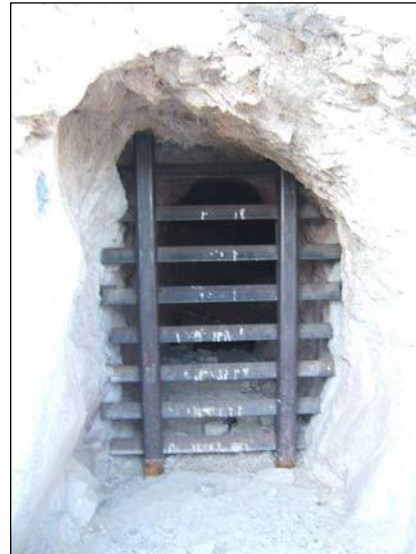
Figure 1.—Example of a gated mine at the Salt Creek Hills Mine near Baker, California.
