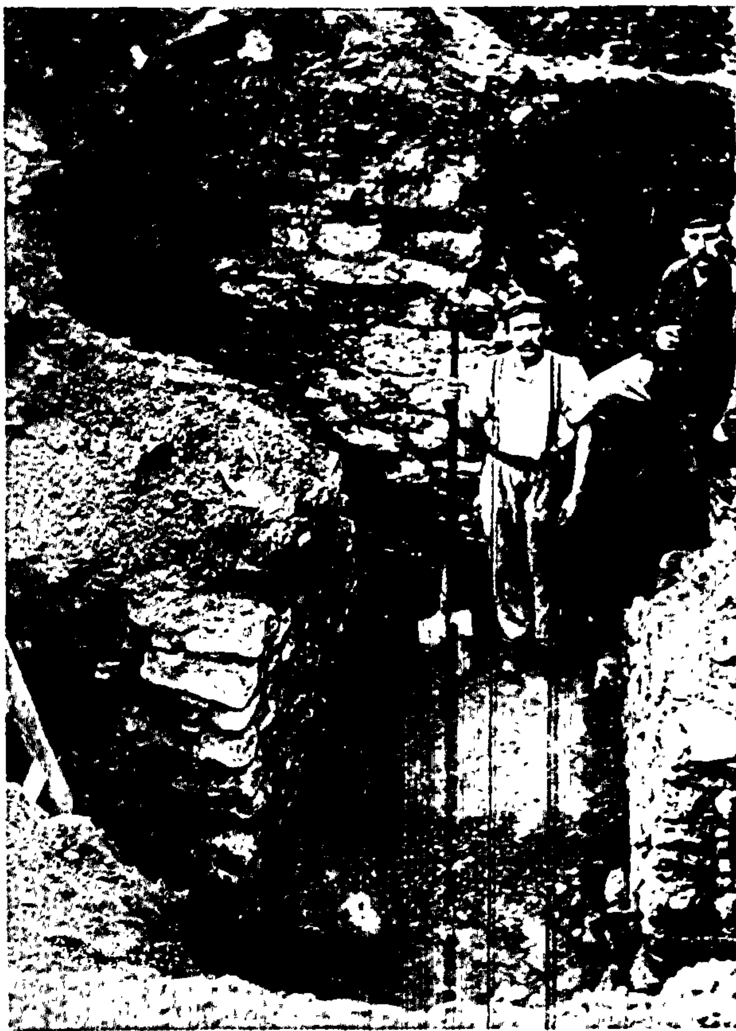
Fig. 3. Gate through the northern wall of the imperial palace in the Carolingian period. Found during street construction in 1906
