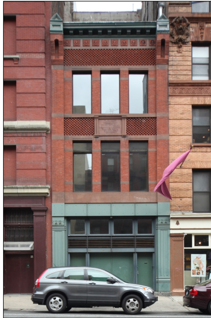
Fire Engine Co. 55 185 Lafayette Street (1886-87 Napoleon LeBrun & Son) Photo by Christopher D. Brazee, 2010
