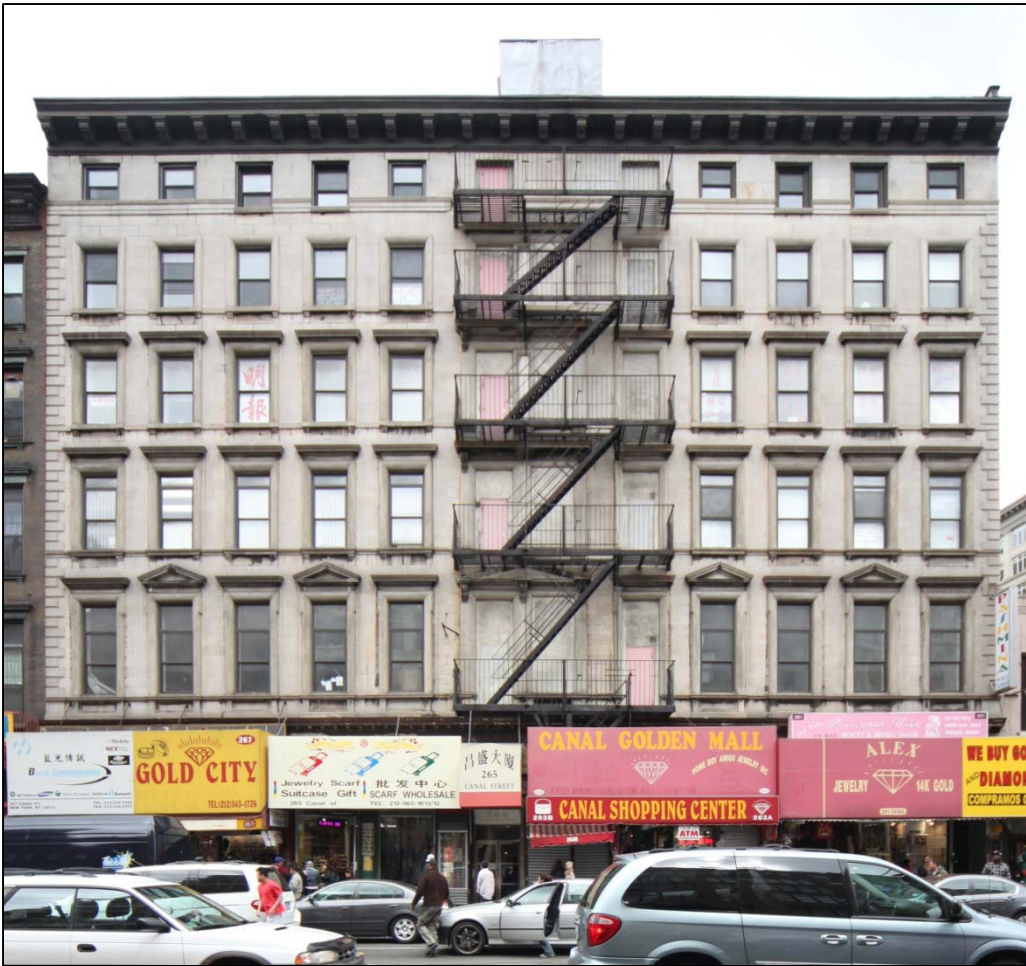
261-267 Canal Street (built c.1853-57 with later alterations), Manhattan Photo by Christopher D. Brazee, 2010
