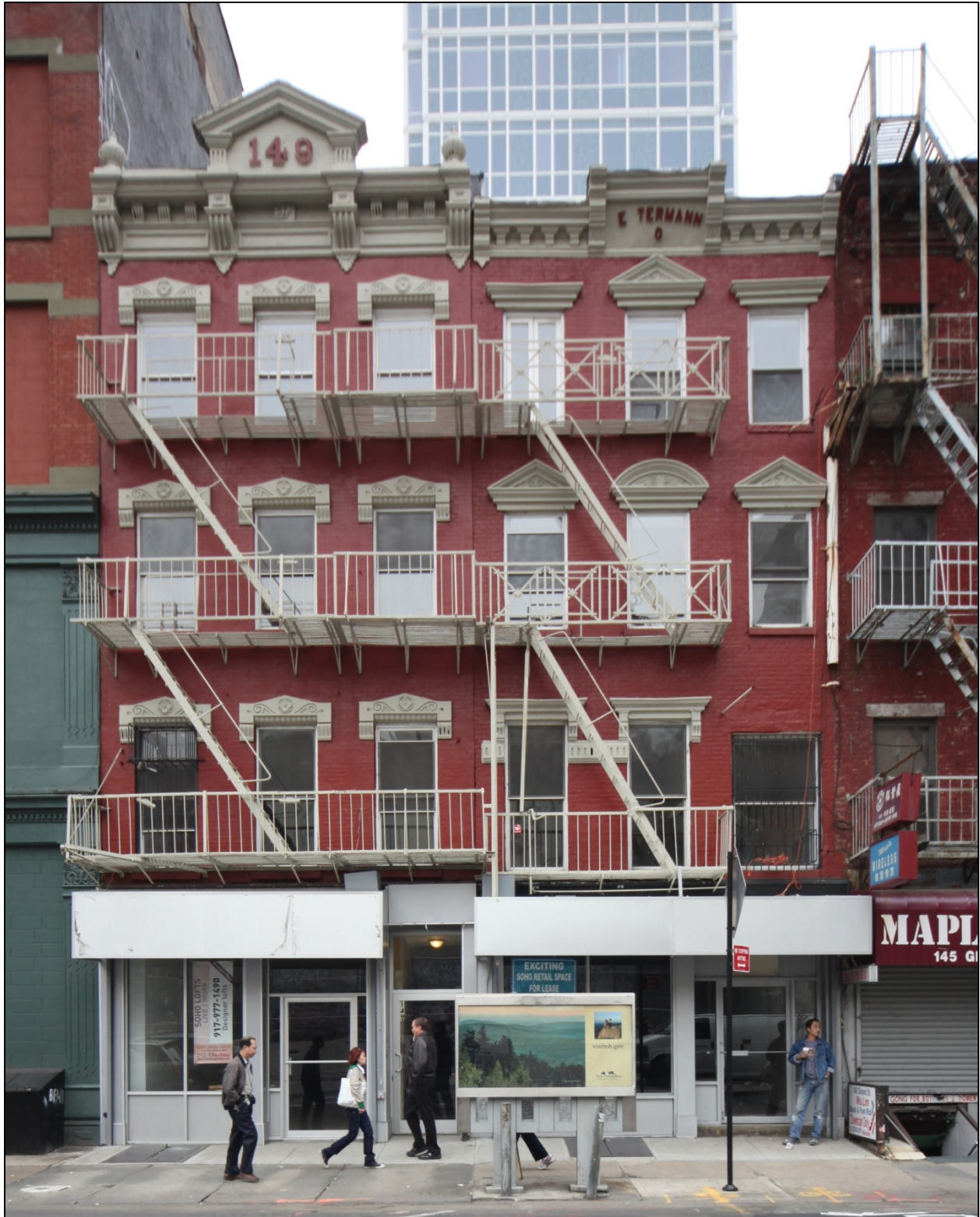
147 and 149 Grand Street (built c.1821-22 with late 19 th century alterations), Manhattan Photo by Christopher D. Braze, 2010
