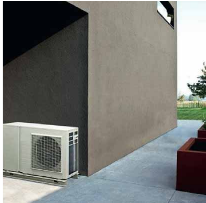
❖ Air/water heat pump (outdoor unit)
