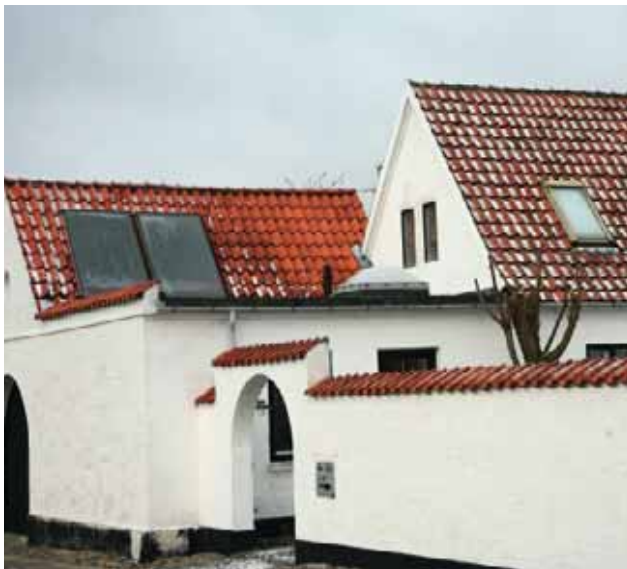
Examples of flat plate collector installations
