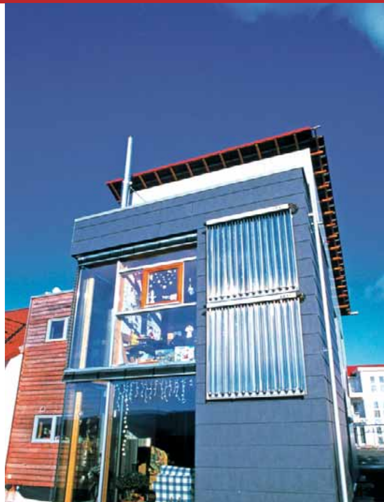
Examples of vacuum tube collector installations
