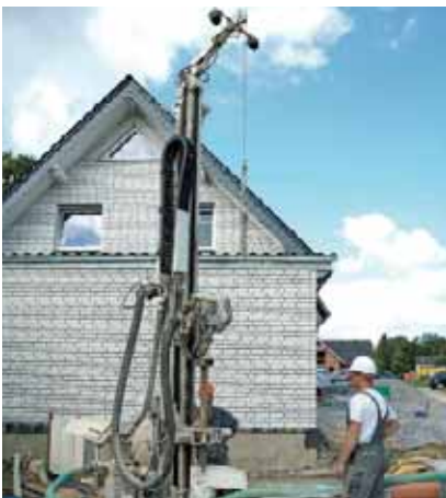
❖ Bore-hole for geothermal heat exchanger
