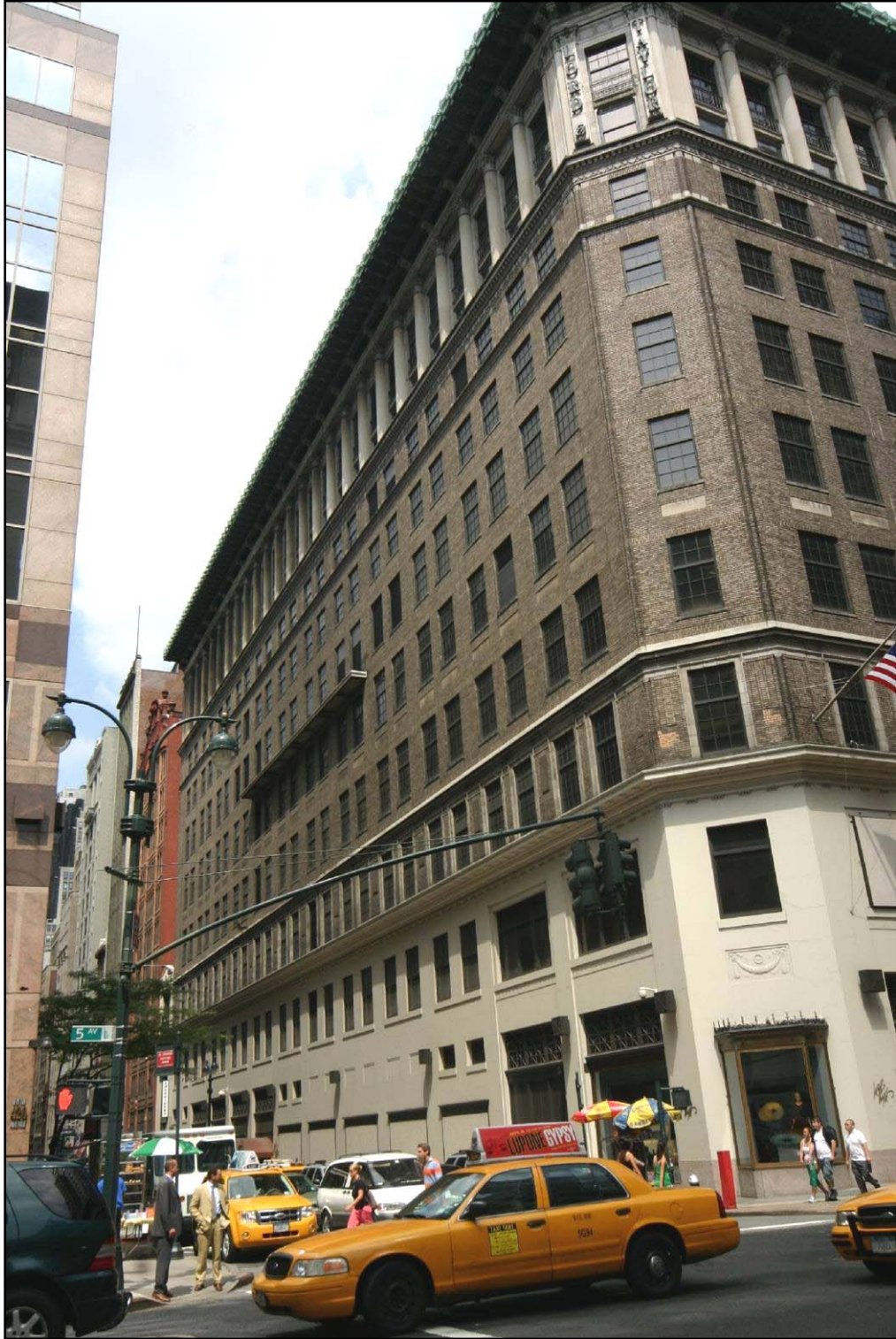
Lord & Taylor Building, West 38 th Street façade Photo: Carl Forster
