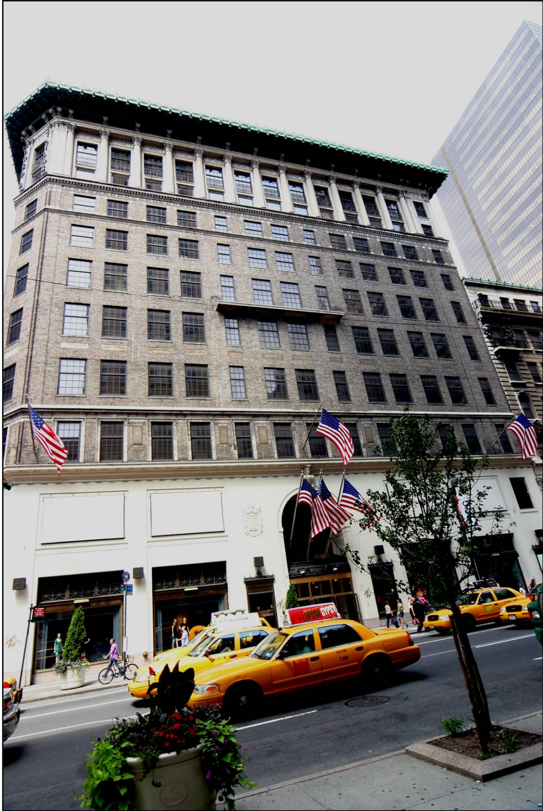
Lord & Taylor Building, Fifth Avenue façade Photo: Carl Forster
