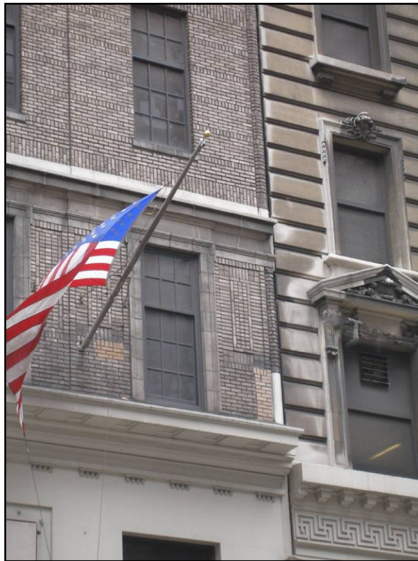
Lord & Taylor Building , façade details Photos: Carl Forster (above), Marianne Percival (below)
