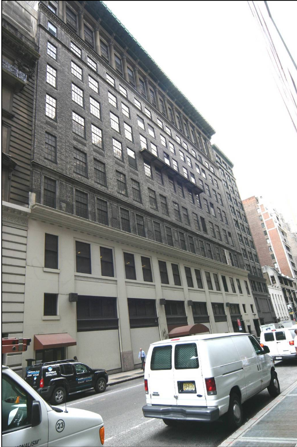
Lord & Taylor Building, West 39 th Street façade Photo: Carl Forster
